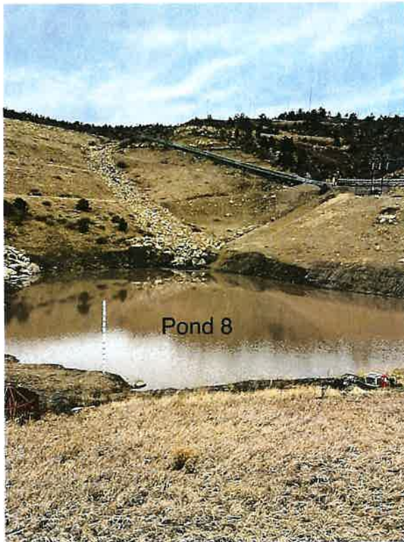
East Drainage of Refuse Disposal Area
