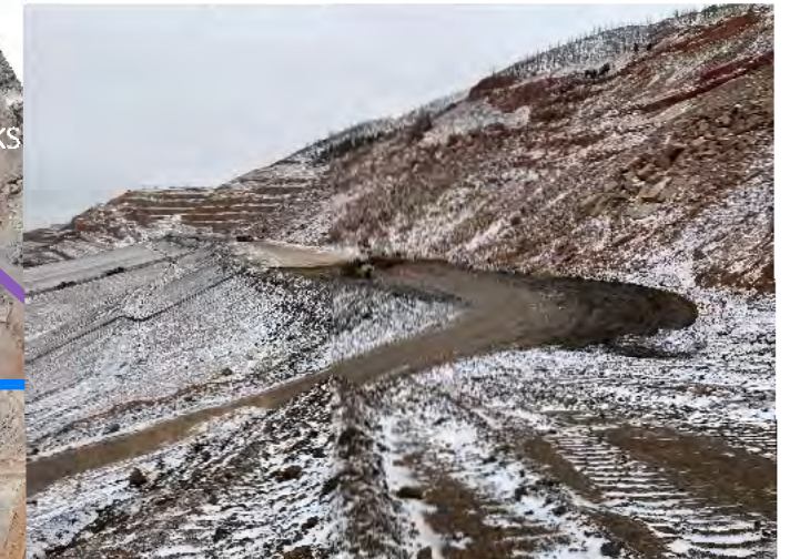
2. Material is placed and compacted on first bench
