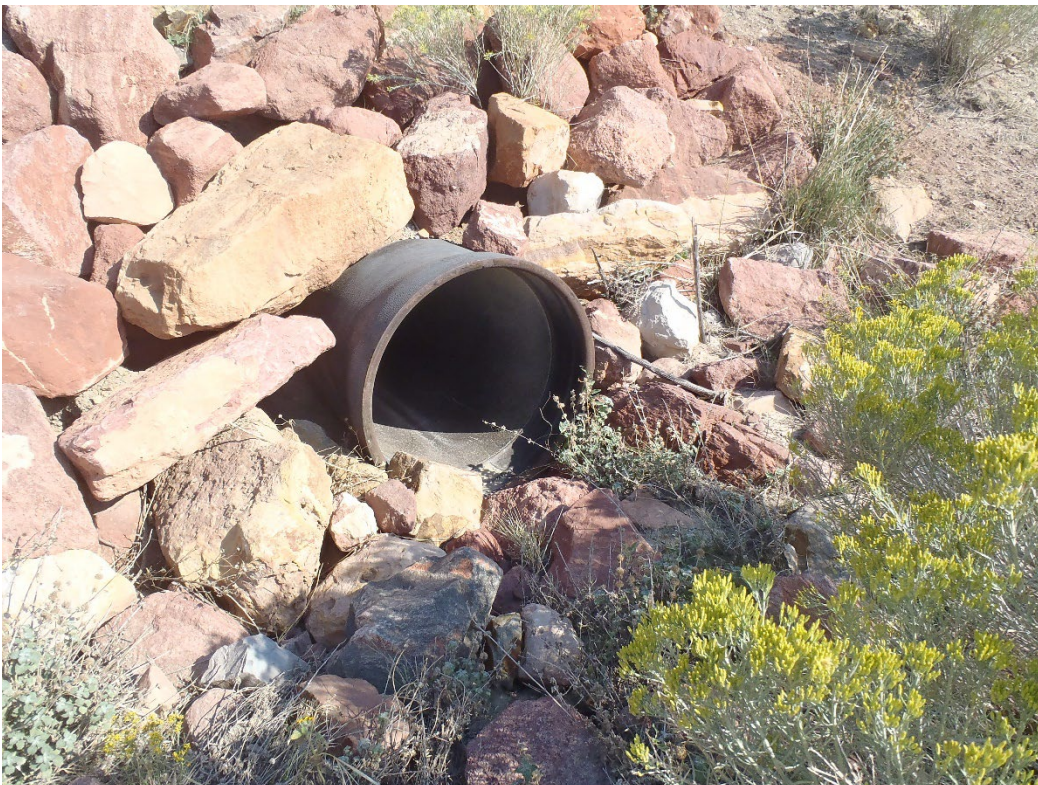
Photo 9. Sedpond culvert (inlet clear).
