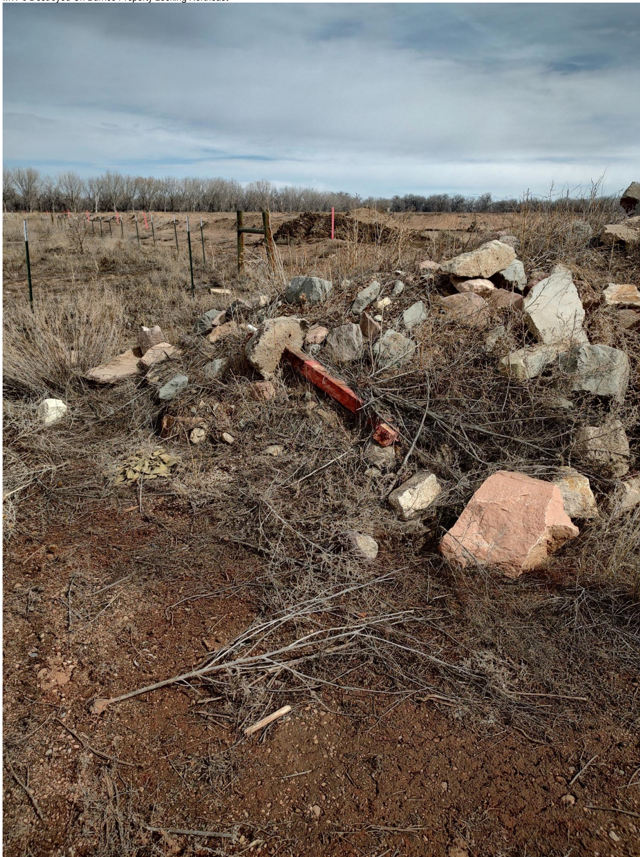
MW-6 Destroyed On Burnco Property Looking Northeast
