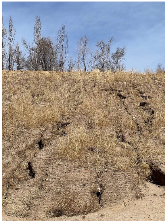
Photo 5. Erosion gullies in central area of buttress
