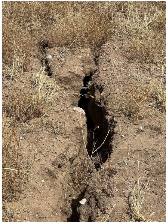
Photo 7. Closeup of erosion gullies near west end of buttress
