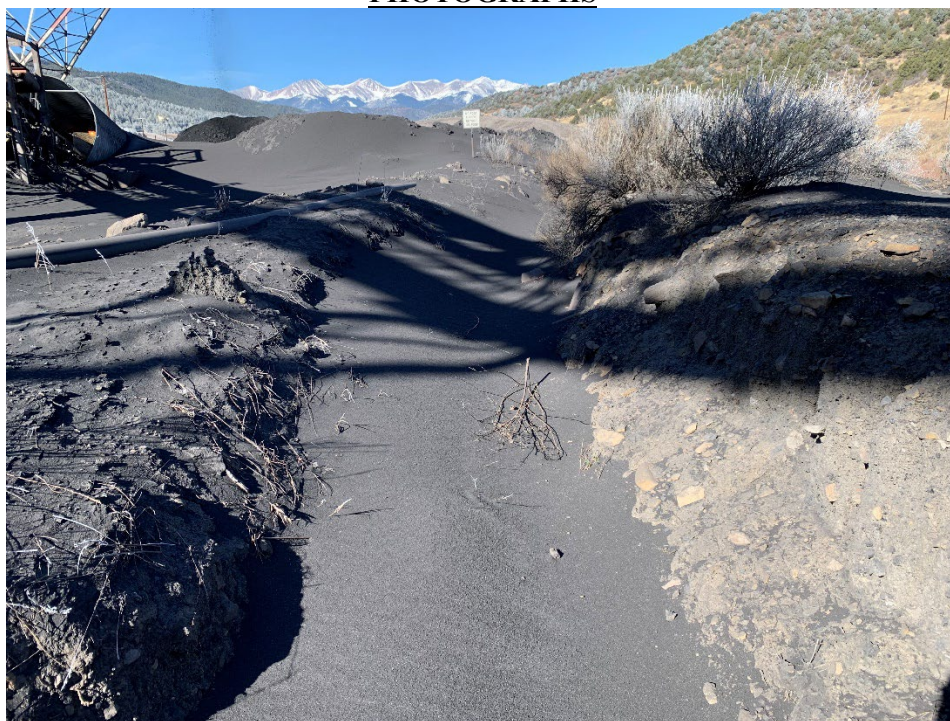
Photo 1 - Ditch D32 filled with coal fines/dust
