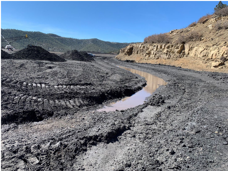
Photo 10 – Standing water in the northeast corner of the RDA
