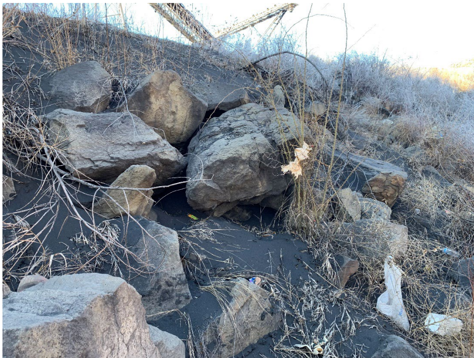
Photo 5 – Coal fines/dust in riprap, elevated conveyor in background (source of dust)
