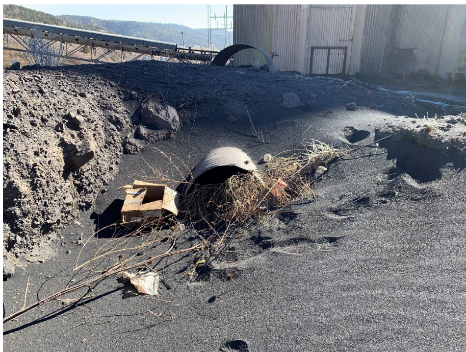
Photo 2 – Culvert C64 obstructed by coal fines/dust
