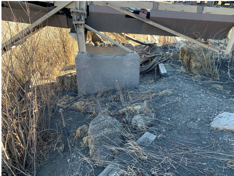
Photo 8 – Sediment control structures under coal refuse conveyor belt
