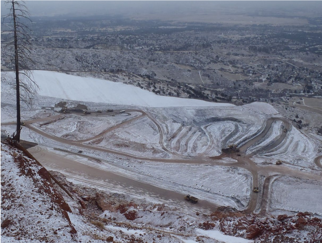
Photo 1. Active excavation of north borrow area (looking north from top of highwall).
