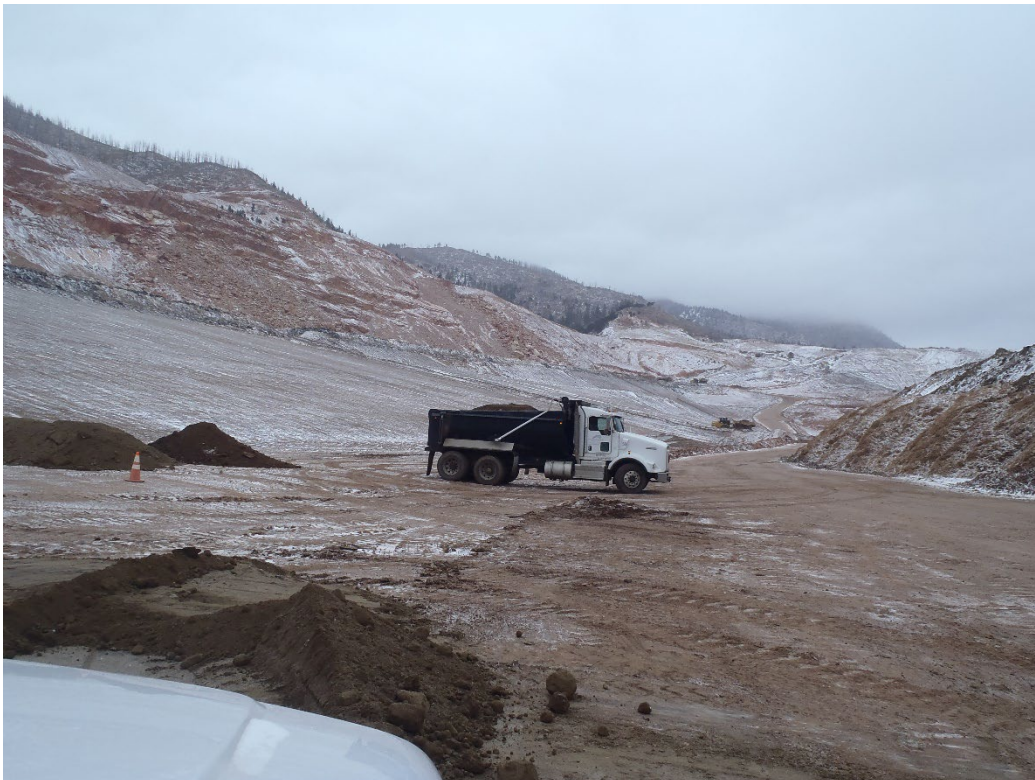
Photo 4. Placing imported topsoil at toe of backfill (looking north).
