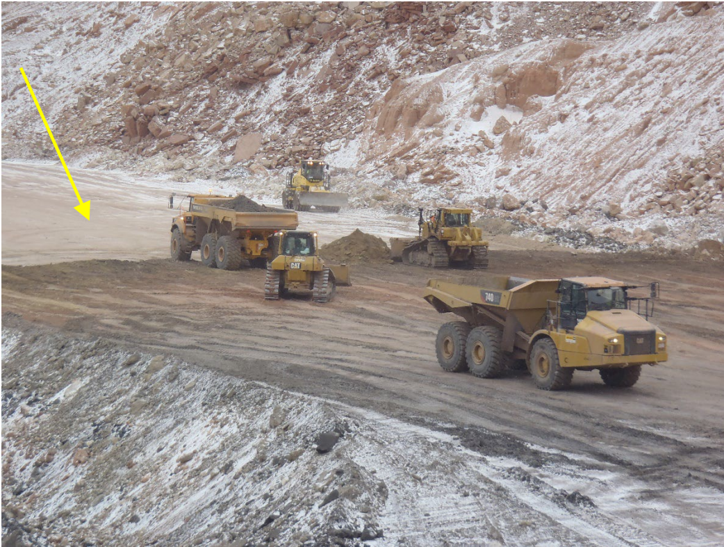
Photo 3. Cleared snow ahead of backfill progressing north to south (looking SW from near north borrow area).
