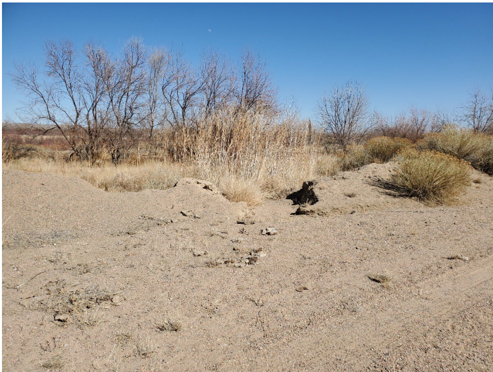
Photo 2: Looking north-west at northern border of western Phase 1 at eroded berm
