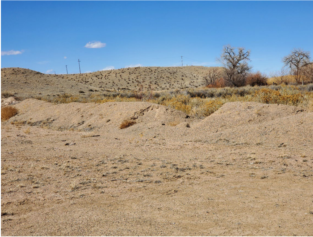
Photo 1: Looking north at northern border of western Phase 1 at eroded berm
