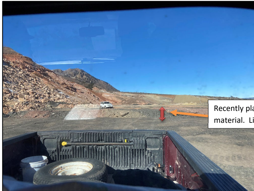
Photo 3 – Main backfill area. Showing one of the lifts of material that the contractor has placed.
