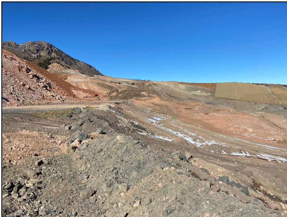
Photo 2 – Fill material is being actively placed in main backfill area.
