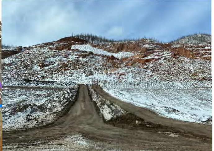
2. Haul road leading to bench work area.
