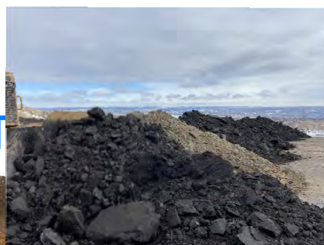
4. Material types are mixed before compaction.
