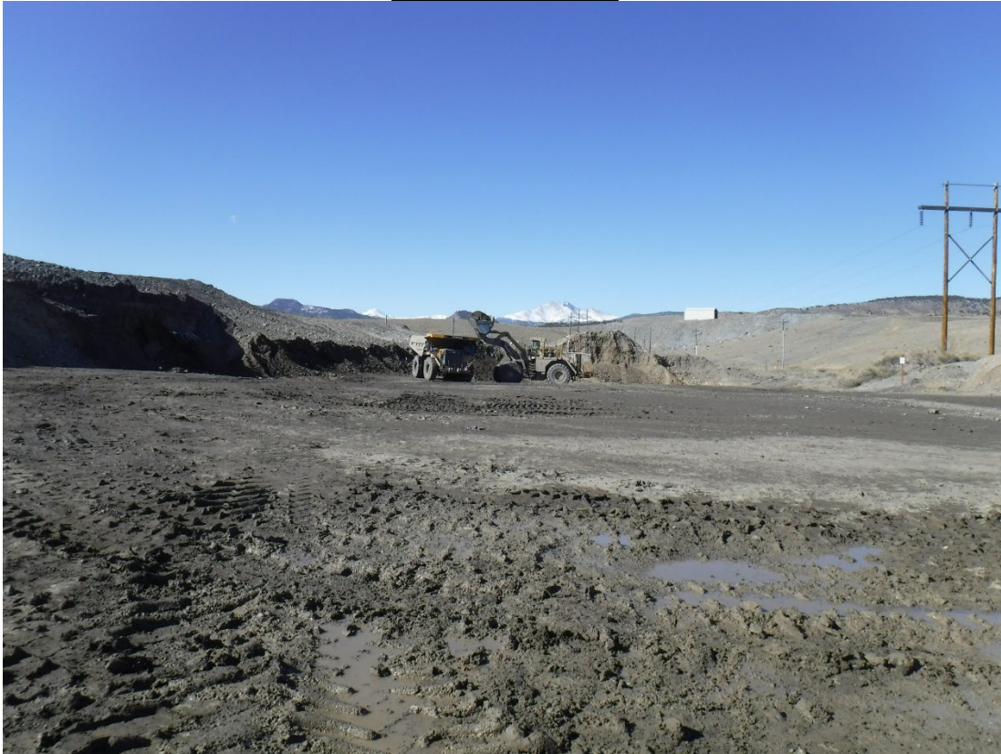
Photo 1: A haul truck being loaded with salvaged overburden material to backfill mine pits
