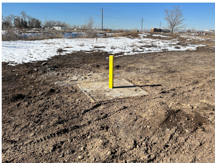
Picture 2 – MW-7 Replacement well
