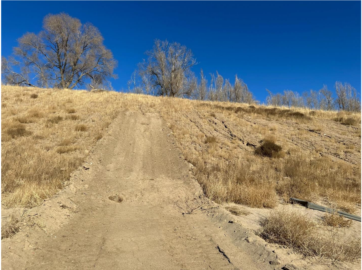
Photo 6. Buttress slope repair looking north from toe, erosion occurring around repair
