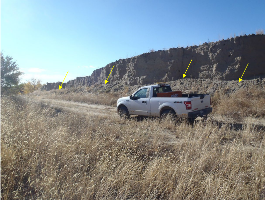
Photo 1. Old wash pond berm – vertical side (note sloughing [arrows], looking south).
