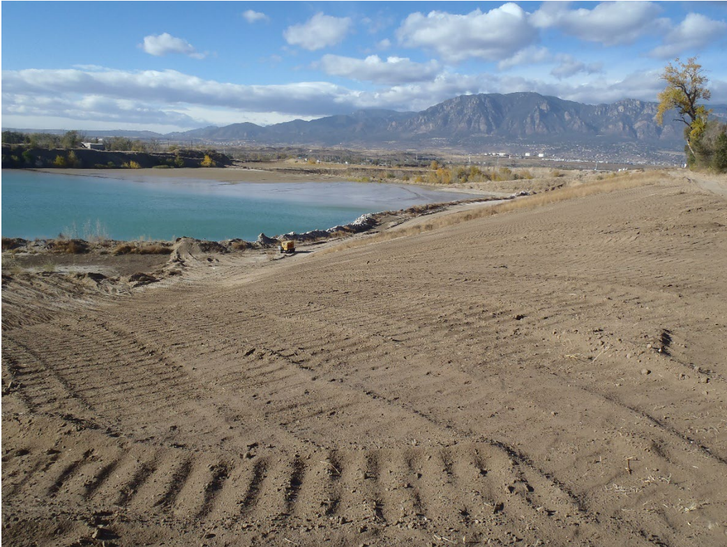
Photo 7. Flattened highwall between Fountain Mutual Ditch and new wash pond (Looking SW).
