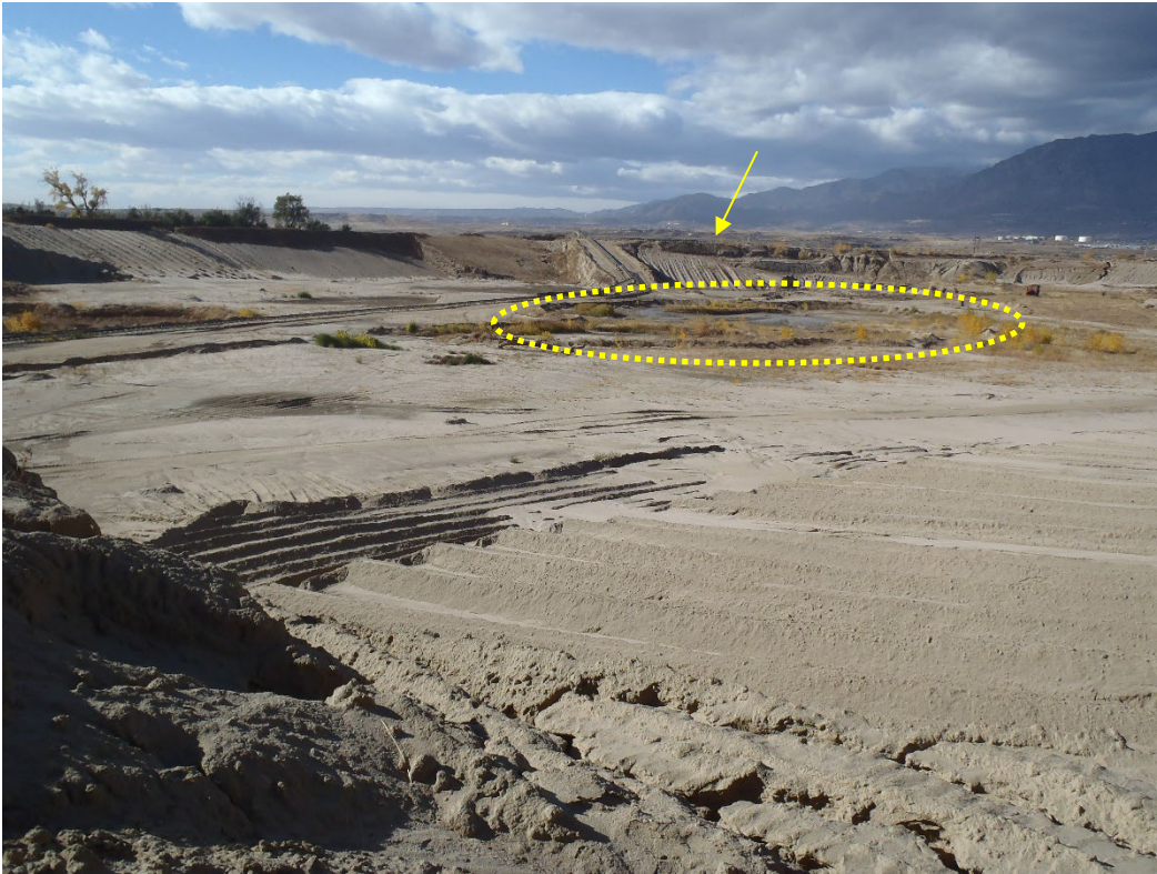
Photo 3. Main pit: standing water [circled] and highwall flattening [arrow] (looking SW from east end).
