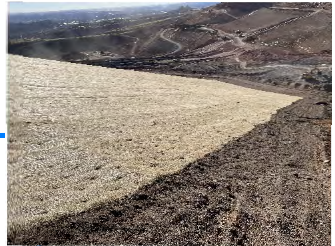
3. Erosion control installed on north borrow slope
