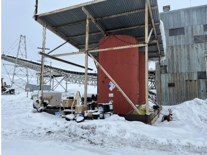
Photo 1: Improper storage of diesel fuel materials, buckets located outside of secondary containment structure.
