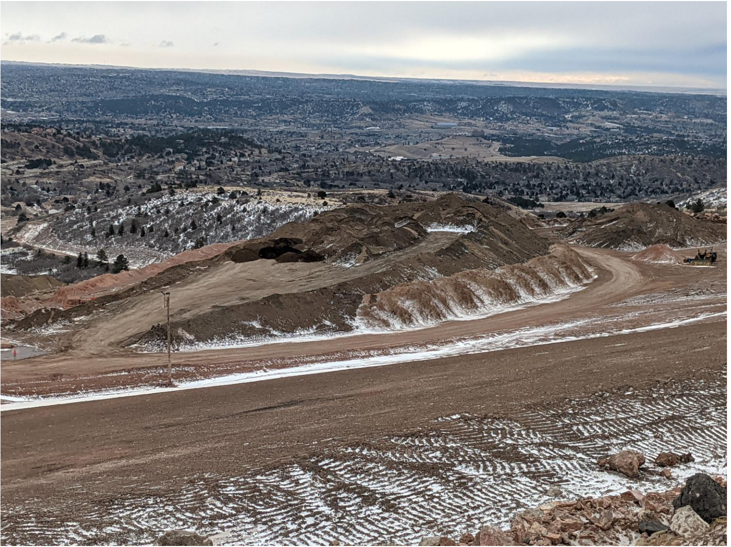
Topsoil stockpiling.
