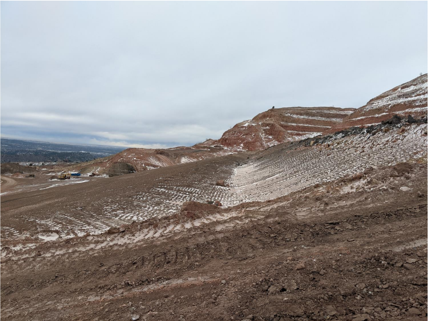
Bench transition of buttress.
