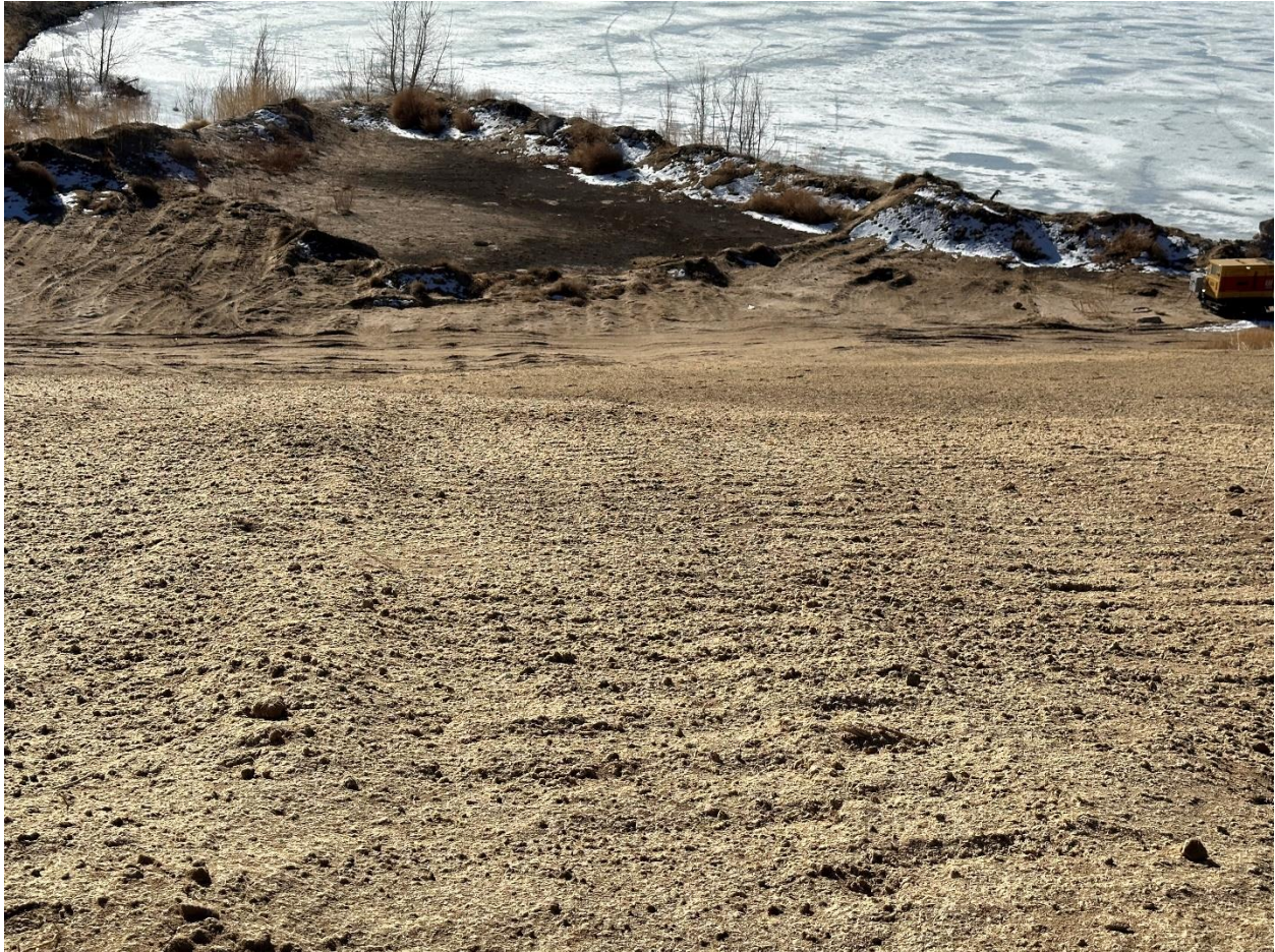
Photo 5. Buttress slope eastern portion with seed
