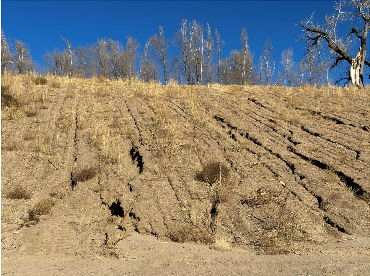
Photo 7. Buttress slope looking north, note evidence of drainage/erosion gullies forming. More sediment near toe
