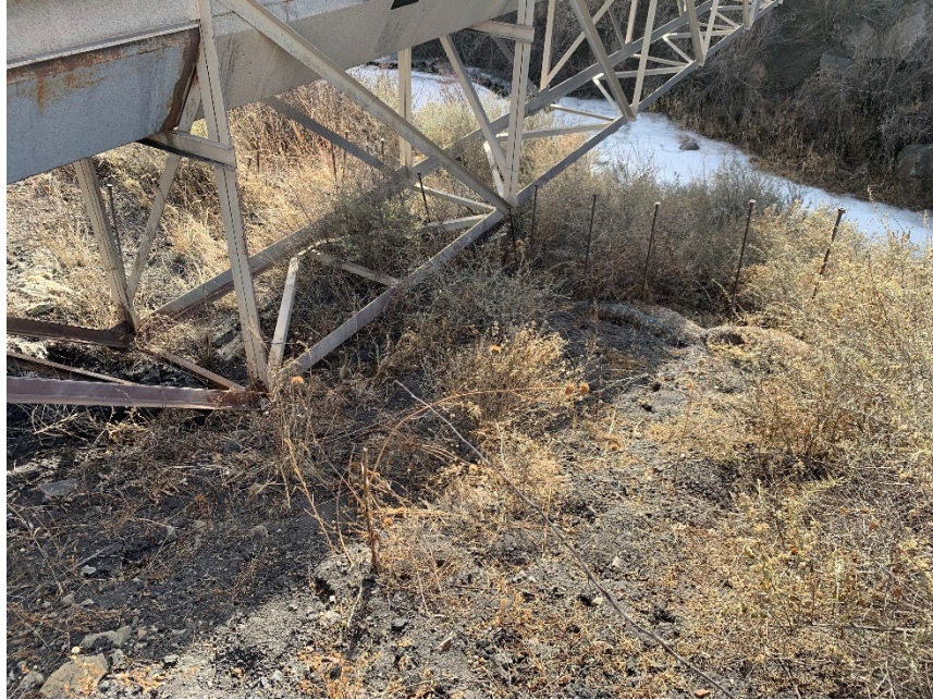
Photo 6 – Silt fence under conveyor that needs to be repaired
