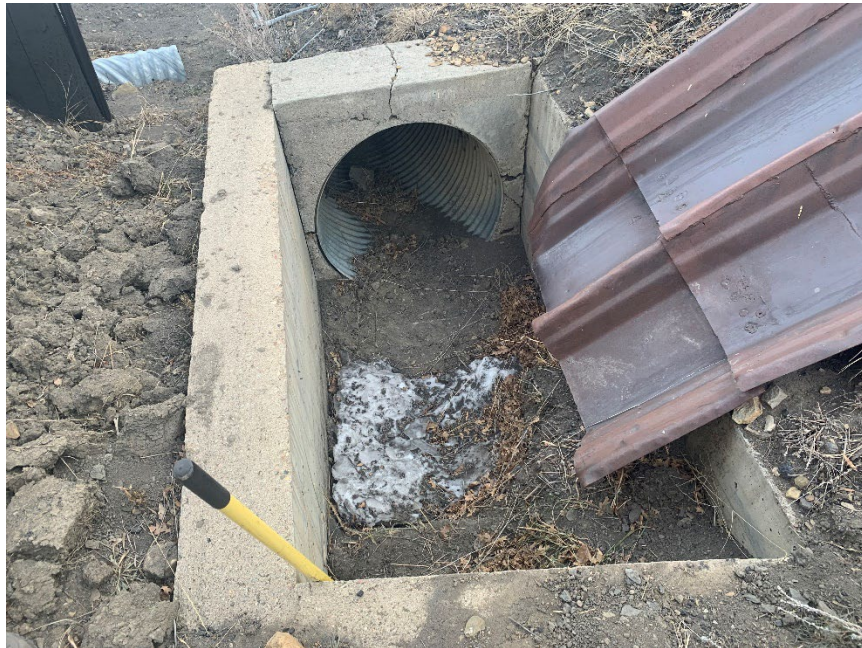
Photo 1 – Clean water diversion box needs to be cleaned
