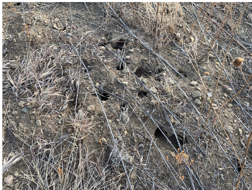
Photo 5 – Rodent holes on the embankment of Pond 1
