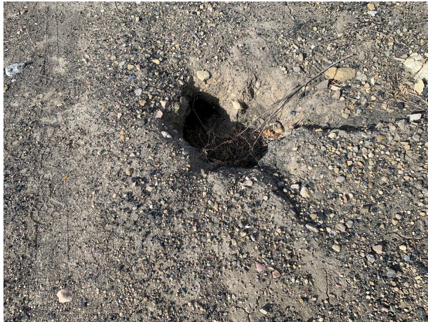
Photo 7 – Hole in access road over the Pond 8 discharge culverts
