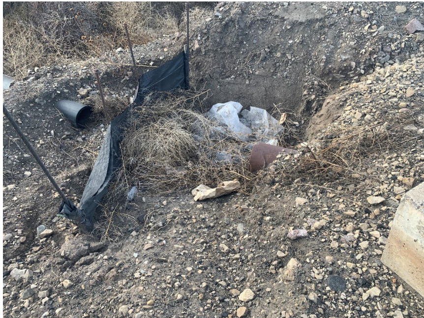
Photo 3 – Debris needs to be removed from sediment trap
