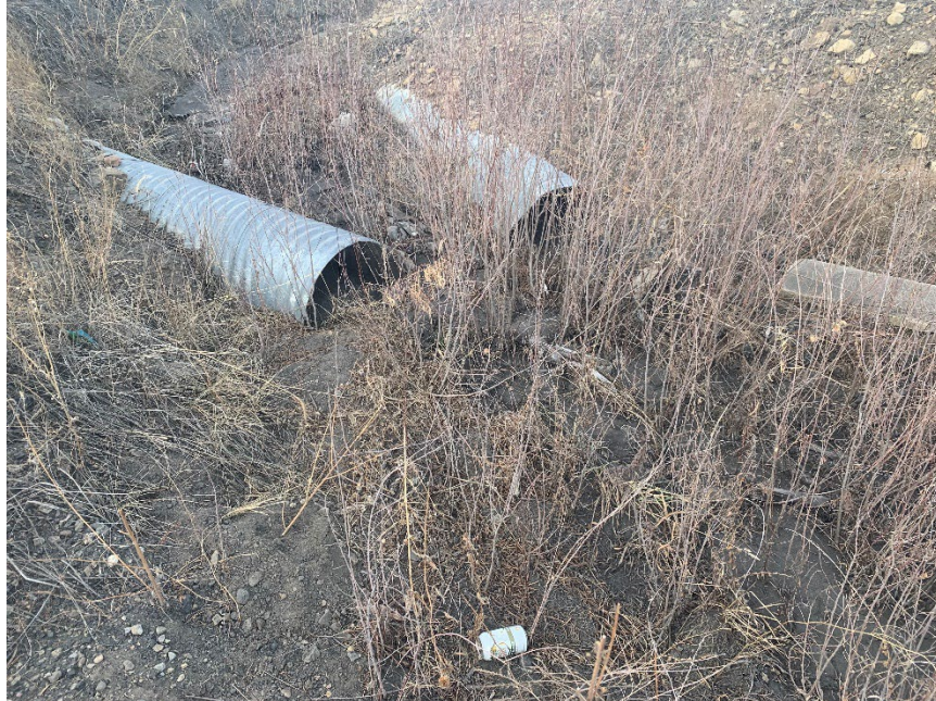
Photo 2 – Willows need to be removed and culverts cleaned
