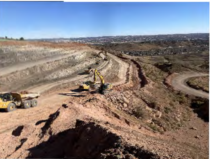
1. Benches in the north borrow area.
