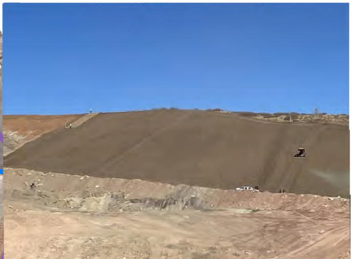
2. Graded slopes in the north borrow area.
