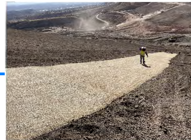
3. Erosion control installed on north borrow slope.
