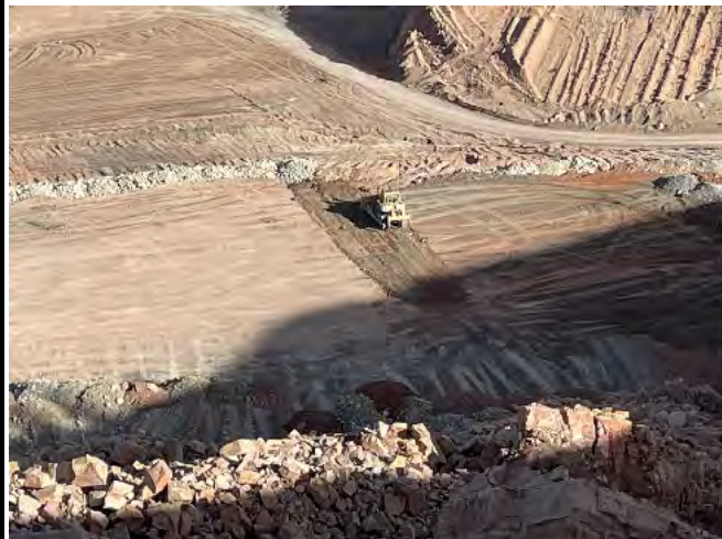
7. Compacted area in the buttress zone.
