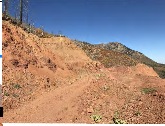
4. Stable granite slopes above landslide.
