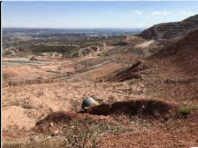
6. View looking south to the buttress fill.
