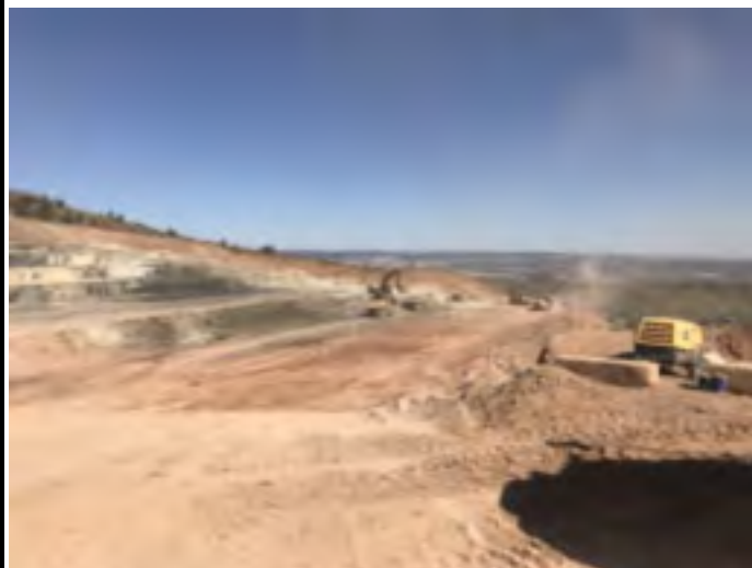
7. Excavator loads haul trucks at shop borrow area.
