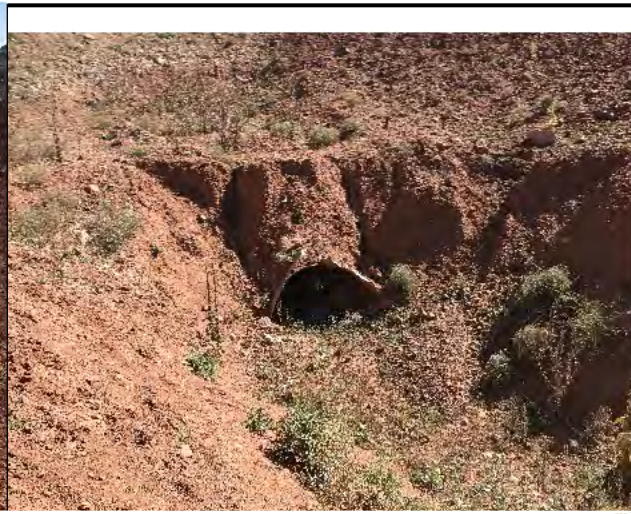
5. Dry above culvert. Note piping for pump if needed.
