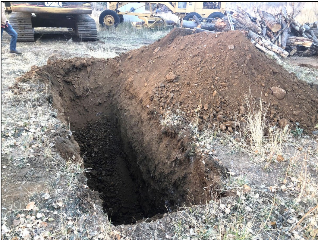
Photo 8. View looking southeast at easternmost soil test pit excavated near base of mesa.
