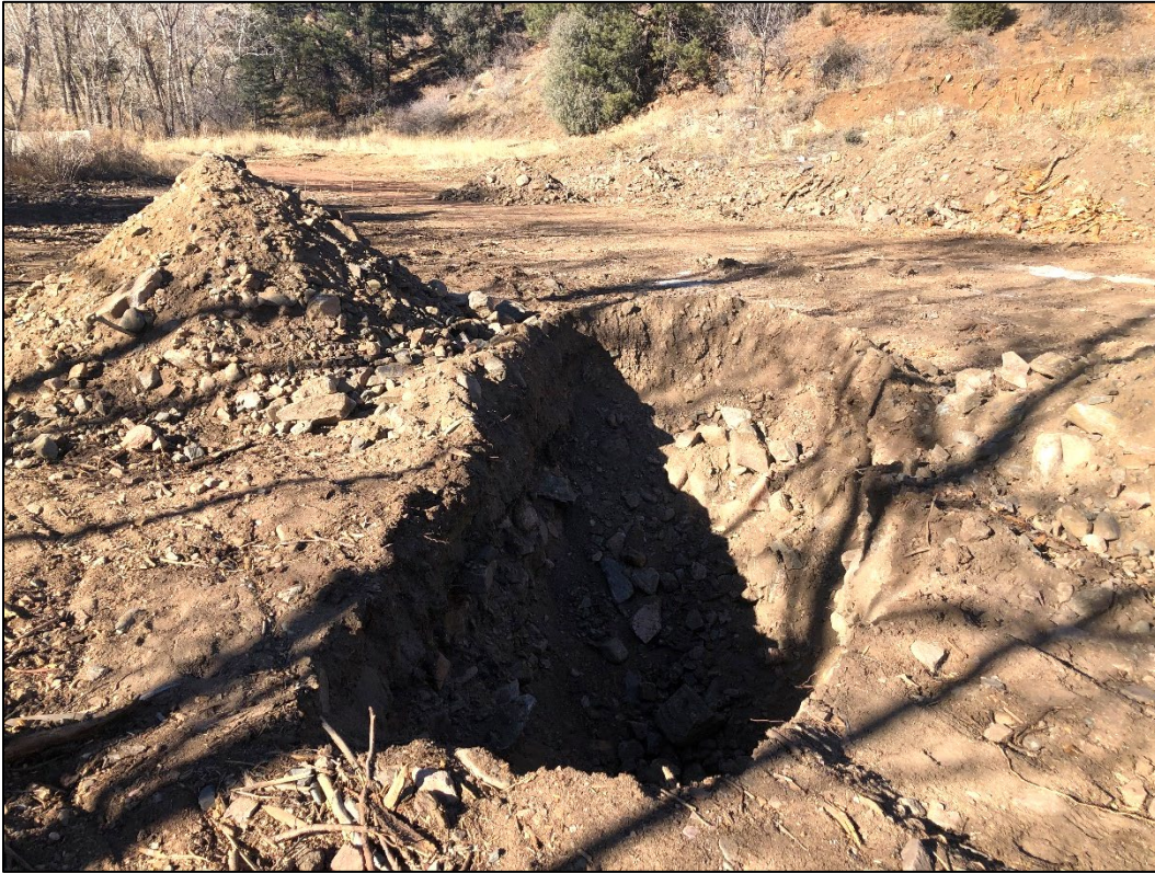
Photo 15. View looking northwest at 2 nd soil test pit (from the west) excavated in storage area located north of creek.
