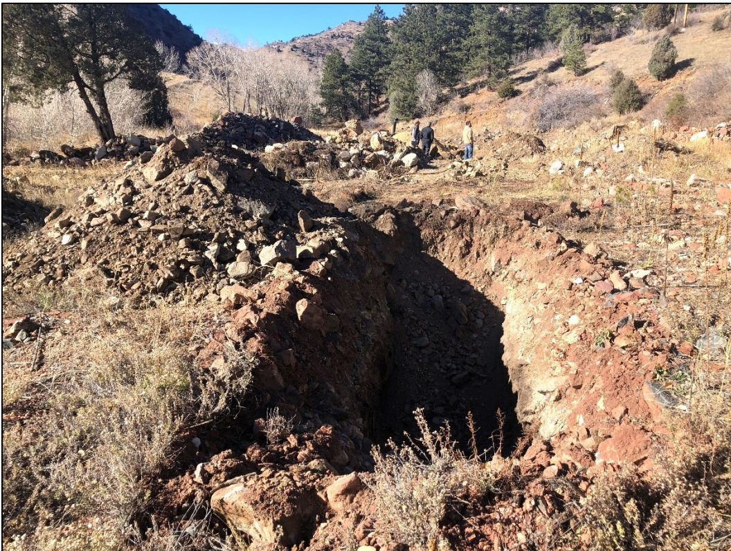
Photo 20. View looking northwest at 4 th soil test pit (from the west) excavated in storage area located north of creek.
