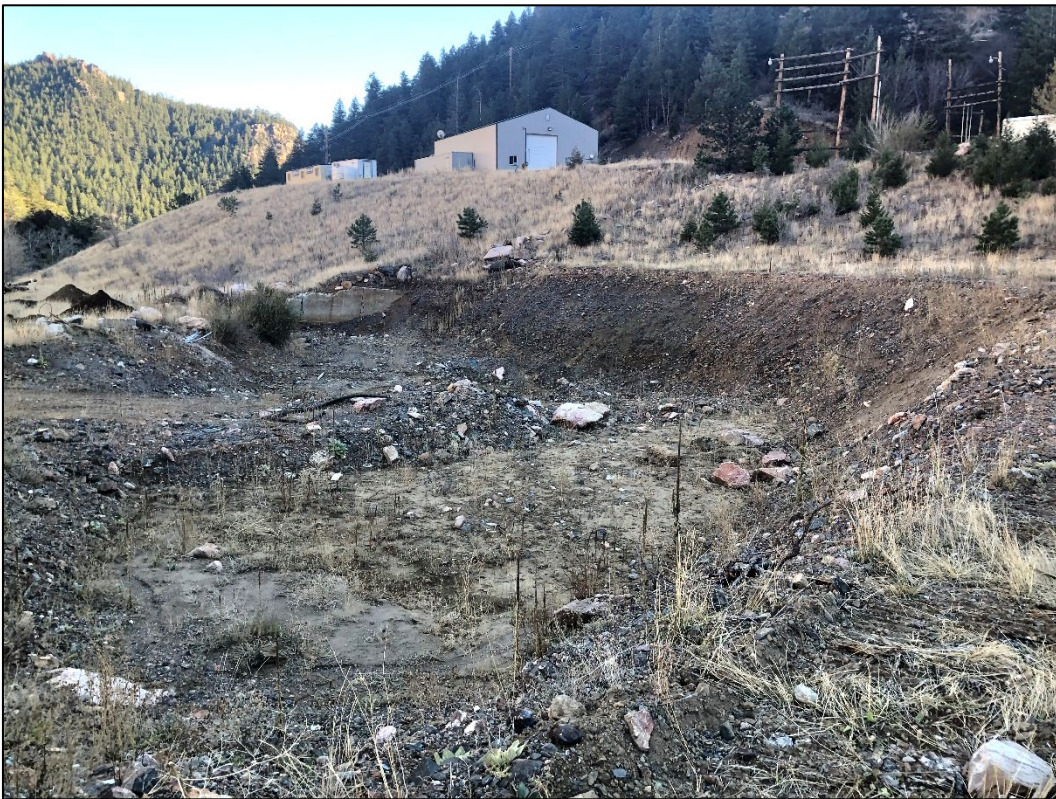
Photo 4. View looking southeast across central excavation area in valley. Note water treatment plant located at top of mesa (in background).
