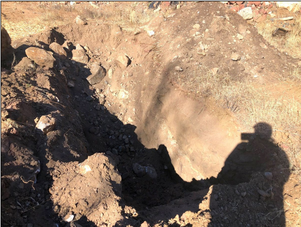
Photo 18. View looking north at 3 rd soil test pit (from the west) excavated in storage area located north of creek.
