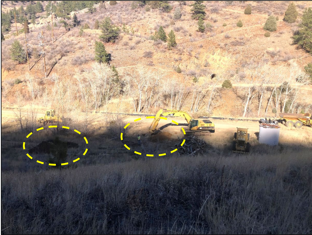
Photo 3. View looking north across valley from top of mesa, showing soil test pits (circled) being excavated near base of mesa during inspection.
