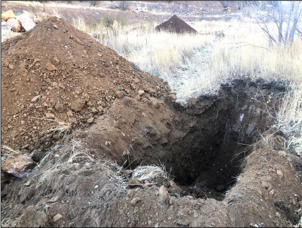
Photo 7. View looking northwest at center soil test pit excavated near base of mesa.
