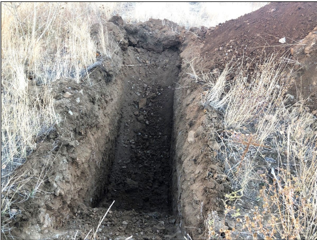
Photo 6. Closer view of westernmost soil test pit excavated near base of mesa.
