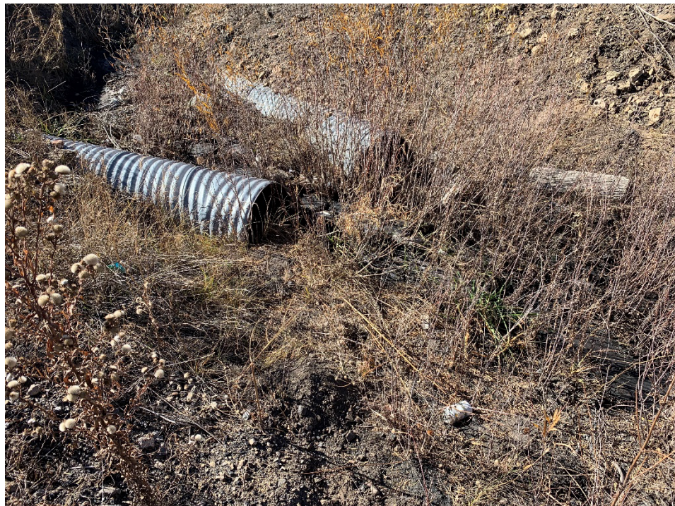
Photo 5 – Willows need to be removed from culvert outlets
