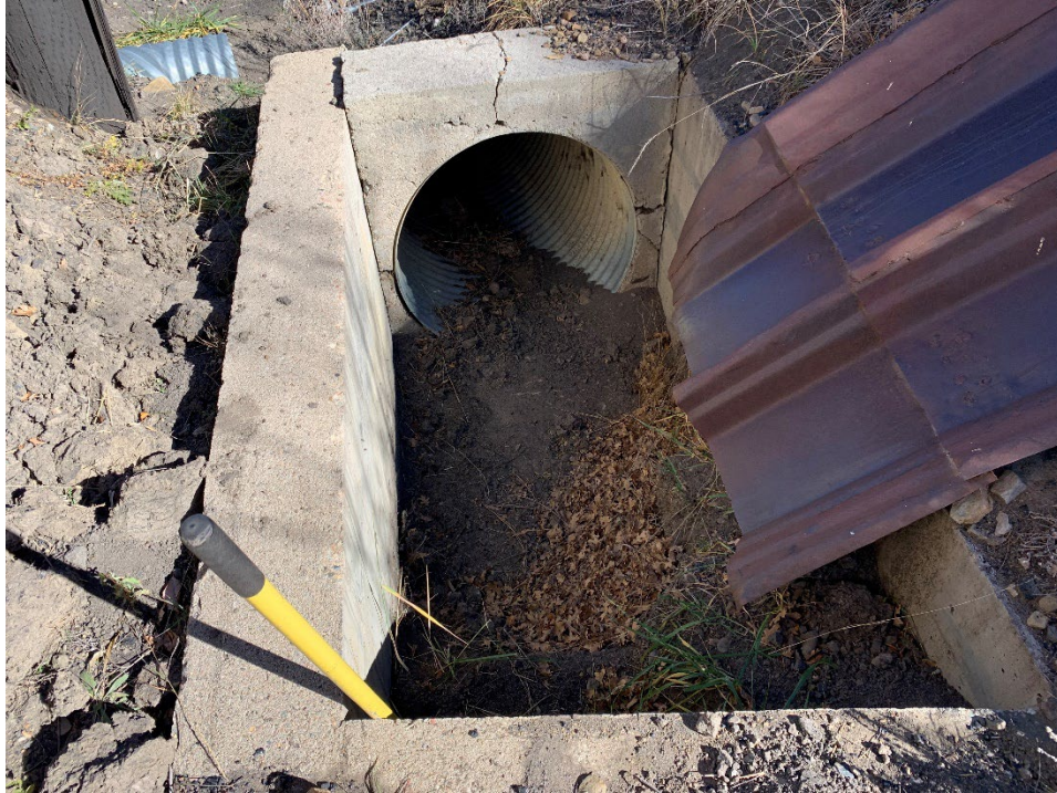
Photo 4 – Clean water diversion box partially cleaned
