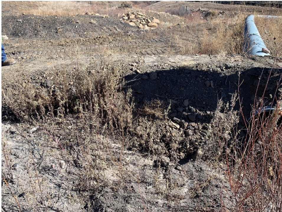
Photo 2 – Sediment basin berm repaired
