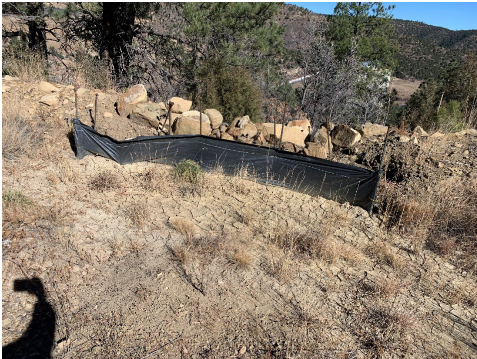
Photo 3 – SAE silt fence in good condition
