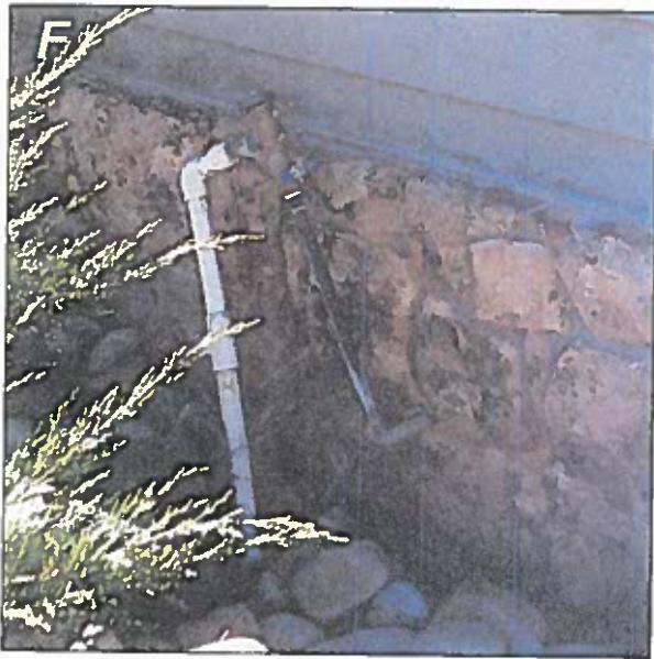
Figure 3-7. F and G , Large wetting events such as broken water mains will cause widespread settlements, ultimately putting the soil of the surrounding area into tension (which is why arcuate cracks form around wetting ponds). In these two photographs, soil is being pulled down and away from the foundation walls. Note the gap along the foundation wall and the distress of the water line into the home. Dangerous conditions occur if natural gas or buried power lines are pulled to the point of rupture.
