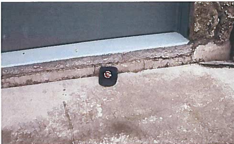
Continued settlement in collapsible soil dropped new town home driveway to a level where vehicles are unable to enter garage. Note leveling slab of concrete on garage floor from previous repair.
