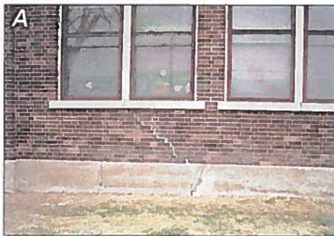
Figure 3-7. A, Typical damage to foundation walls and brickwork from settlement is visible on a school in Canon City.
