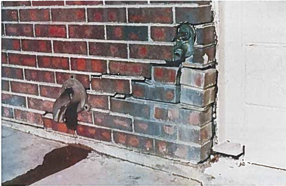
Damage to foundation and mortared brick walls from settlement of collapsible soils. Building in Montrose was demolished shortly after photo was taken. [Photo credit: Buckhorn Geotech]
