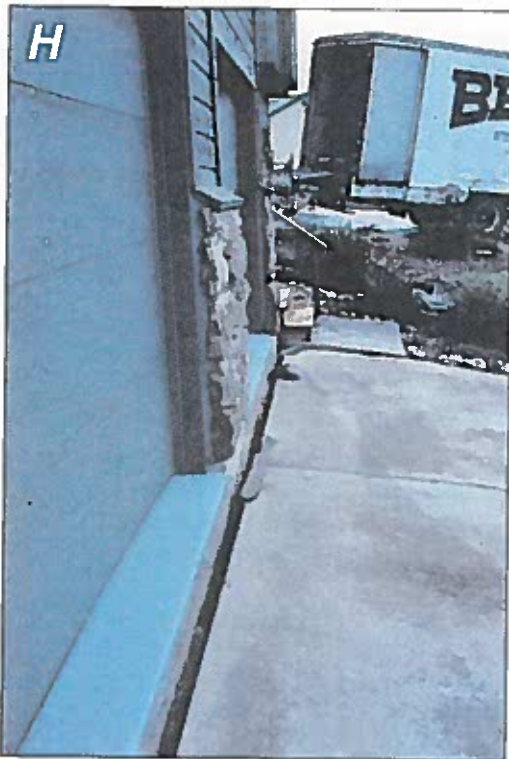
H and I , Large-scale settlement due to a water main break in road (off picture) has pulled this driveway down and away from the residence. This residence was previously underpinned, and a new leveling concrete pad was poured in the garage. The pipe piles were of inadequate depth, and deeper wetting of the collapsible soils caused further distress to the structure. (In I , a baseball hat shows the scale).
