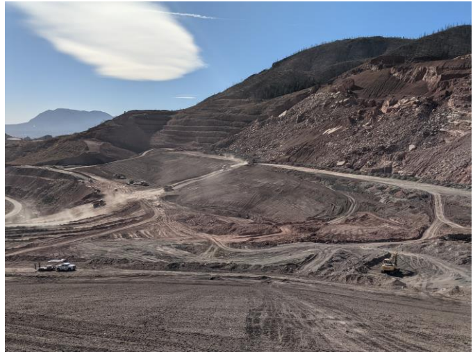
Fill placement at buttress.
