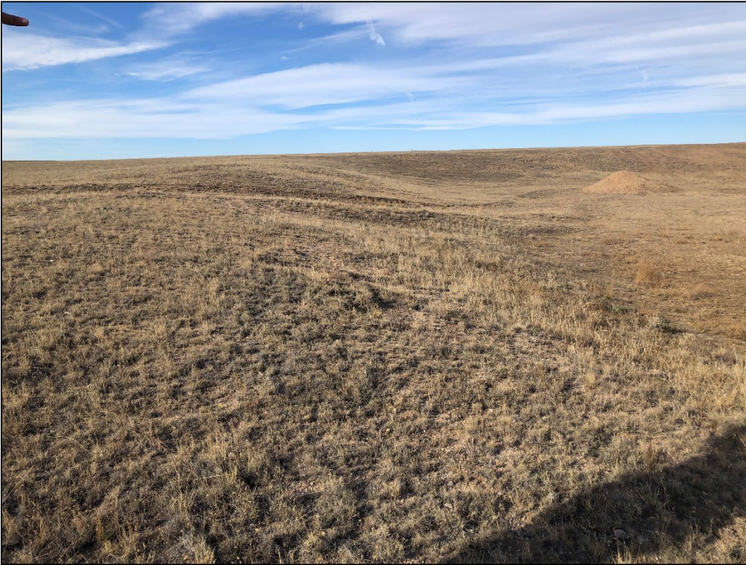
Photo 1. View looking west across reclaimed southern pit wall, showing slopes graded to 3H:1V or flatter with a good grass cover.
