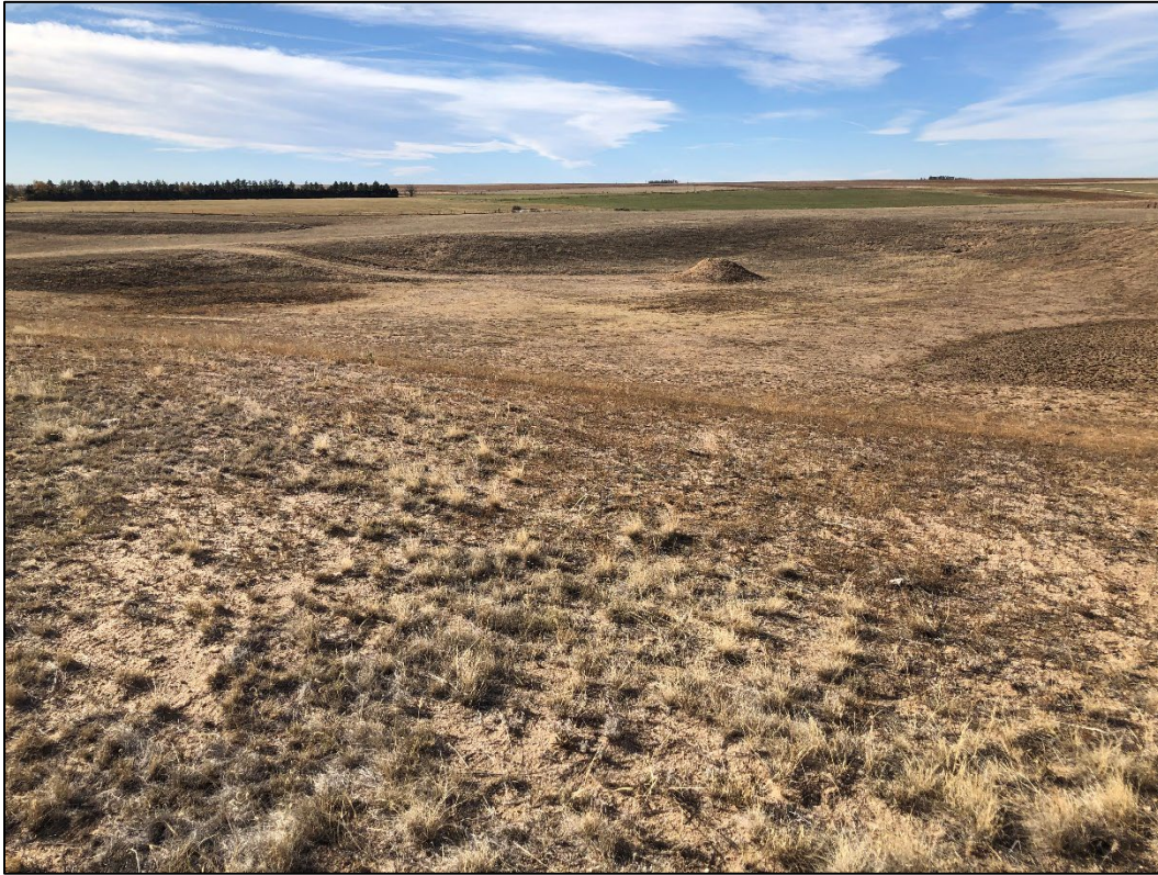
Photo 7. View looking southwest across reclaimed pit, showing slopes graded to 3H:1V or flatter with a good grass cover. Note small gravel pile (at center, right) left on pit floor for landowner use.
