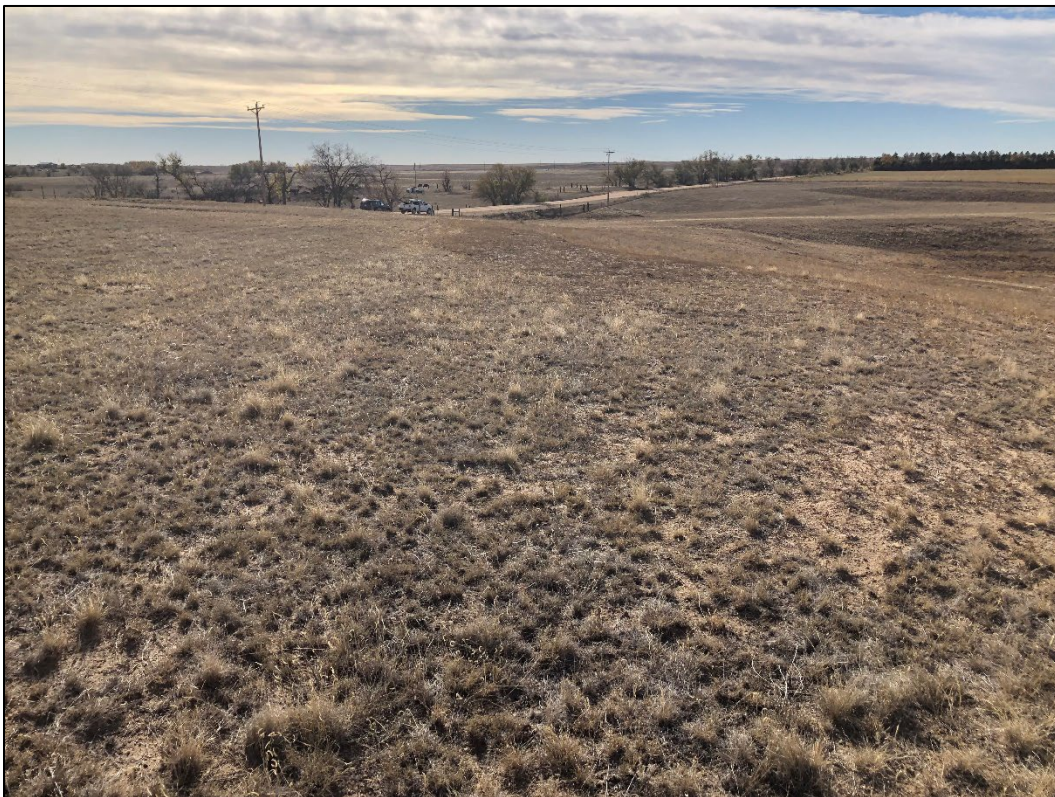
Photo 6. View looking southeast across reclaimed eastern pit wall, showing slopes graded to 3H:1V or flatter with a good grass cover.
