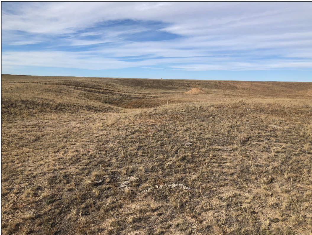
Photo 8. View looking west across reclaimed pit, showing slopes graded to 3H:1V or flatter with a good grass cover.
