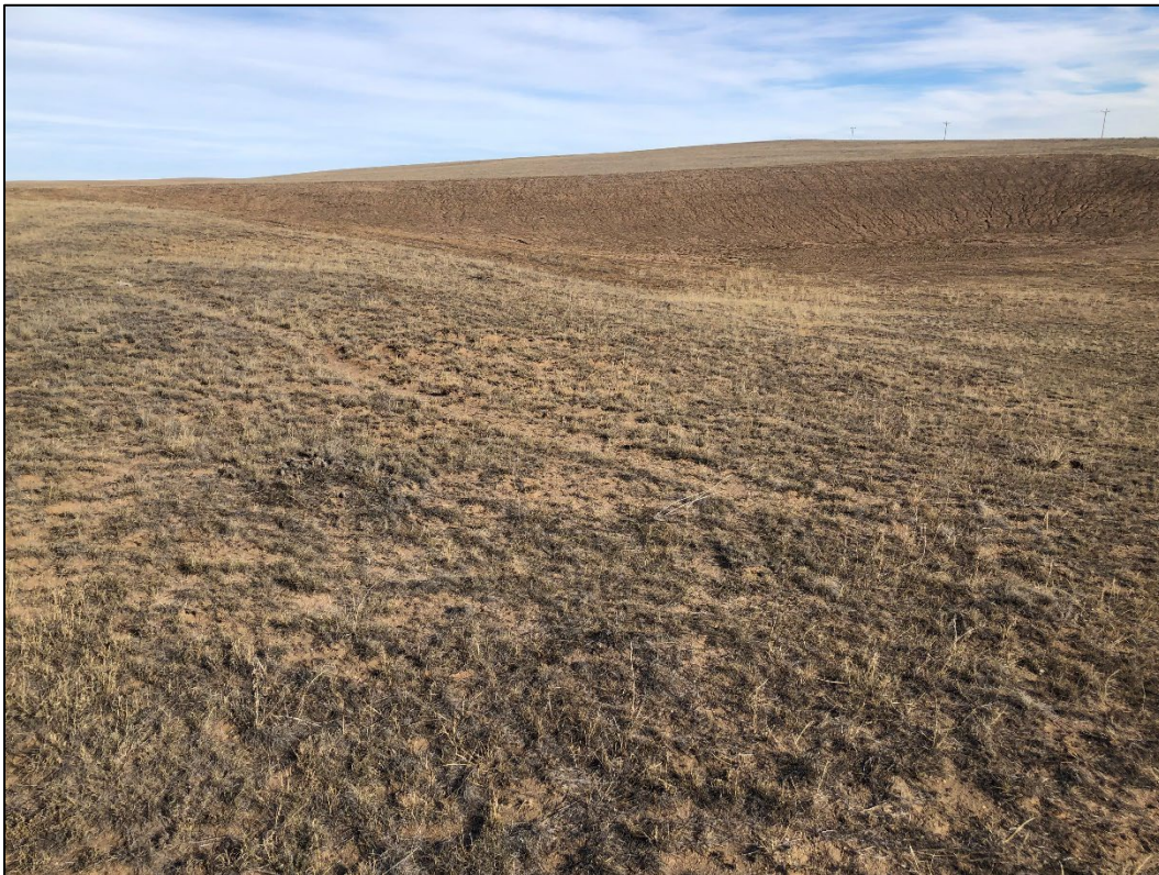
Photo 4. View looking north across reclaimed western pit wall, showing slopes graded to 3H:1V or flatter with a good grass cover.
