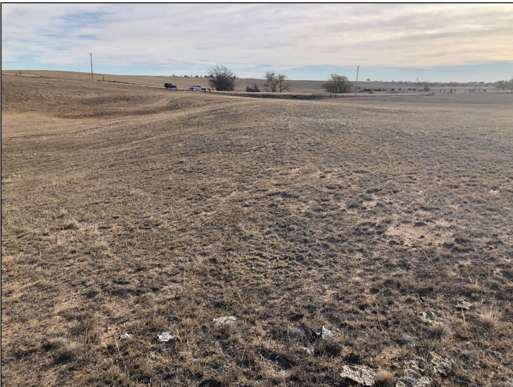
Photo 2. View looking east across reclaimed southern pit wall, showing slopes graded to 3H:1V or flatter with a good grass cover.
