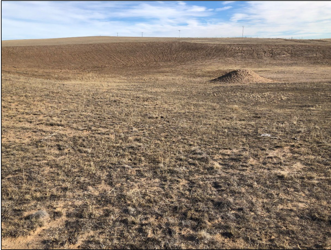
Photo 3. View looking north across reclaimed pit, showing slopes graded to 3H:1V or flatter with a good grass cover. Note small gravel pile (at right) left on pit floor for landowner use.
