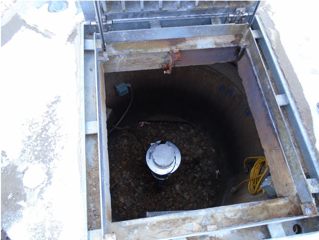
View of the permanent mill water return line valve
