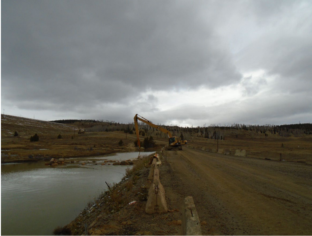
View of the north seep canal dredging operation
