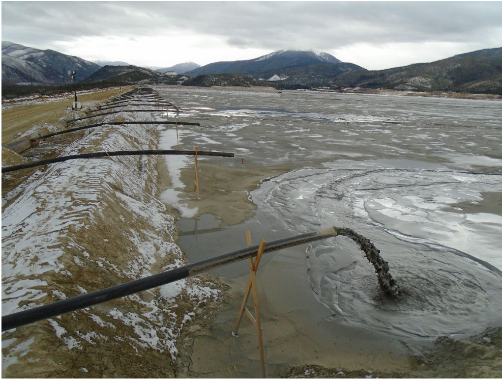
View of spigot deposition in Cell 7 on 1-Dam
