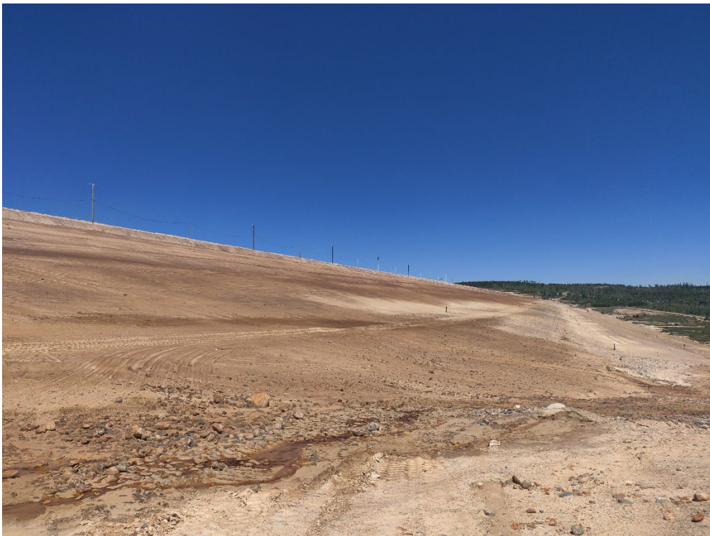
View of the coherex application on the face of 1-Dam
