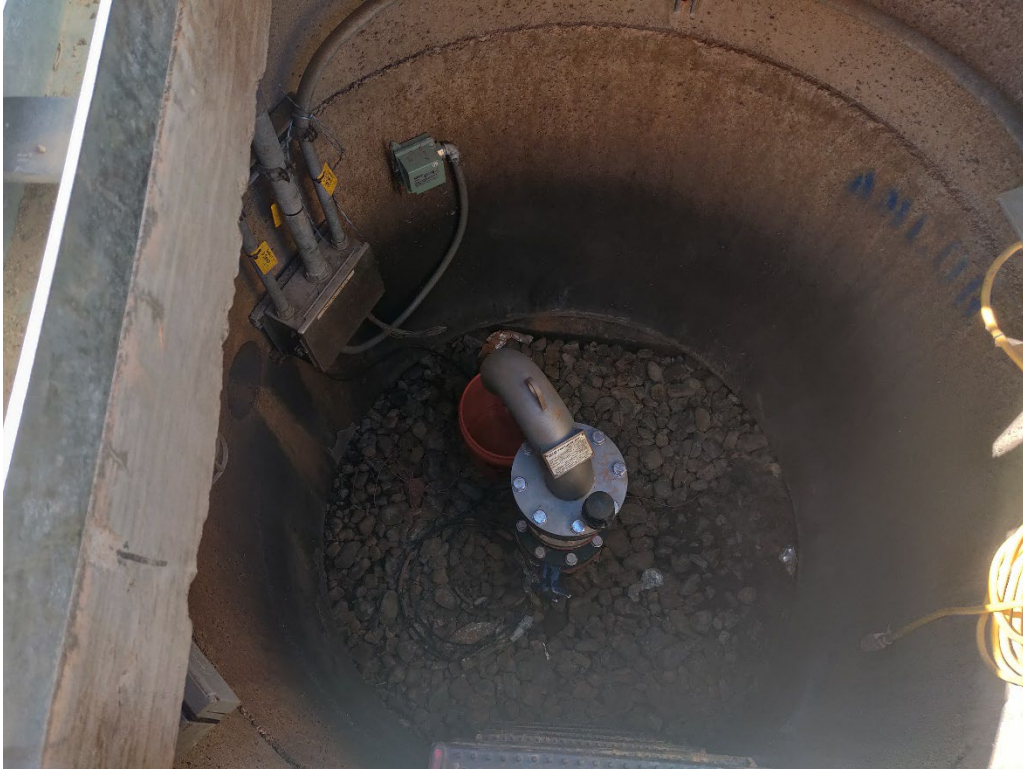
View of the temporary return line valve
