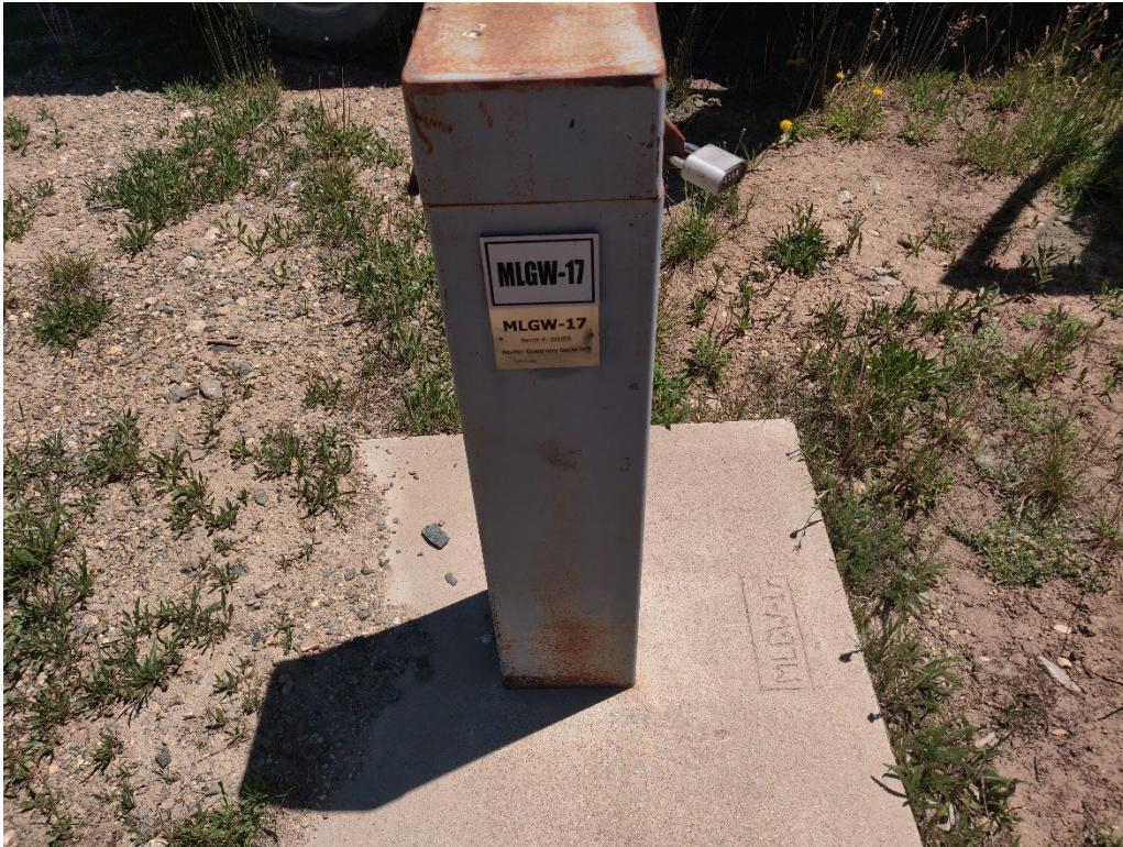
View of MLGW-17 well casing and sign
