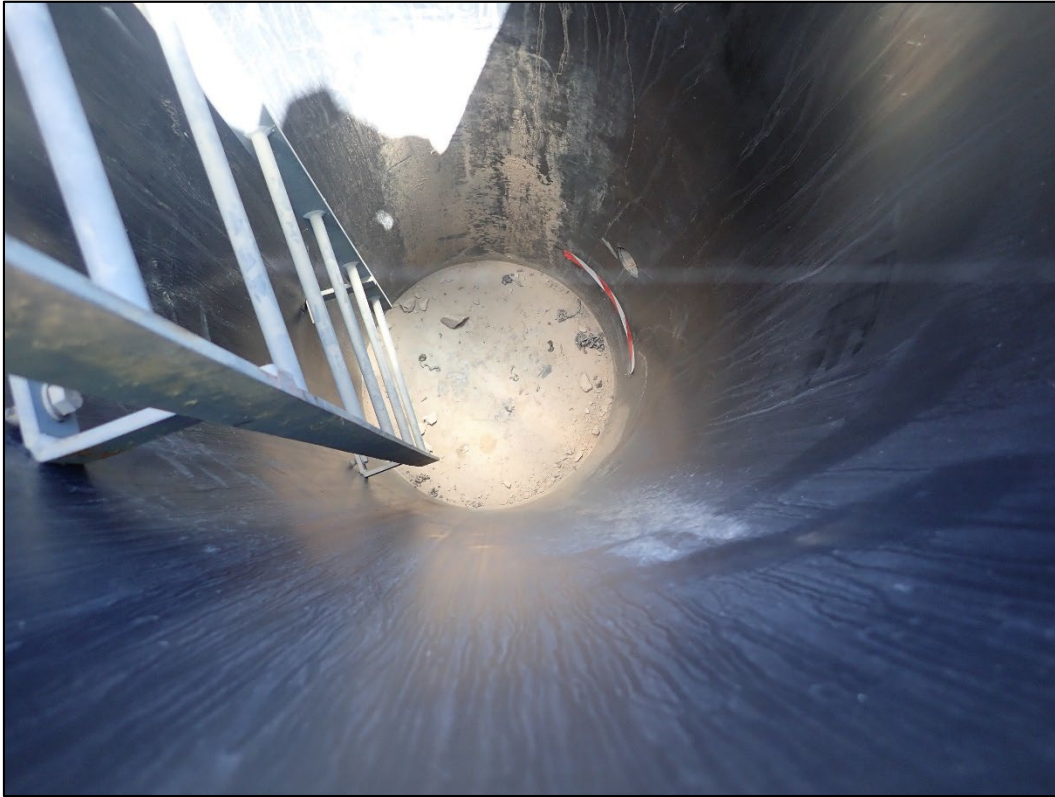
Photo 13. VLF2 LDS 3; looking down.
