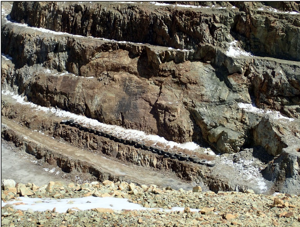
Photo 8. Truck tire berm below South Cresson bench failure; looking north.
