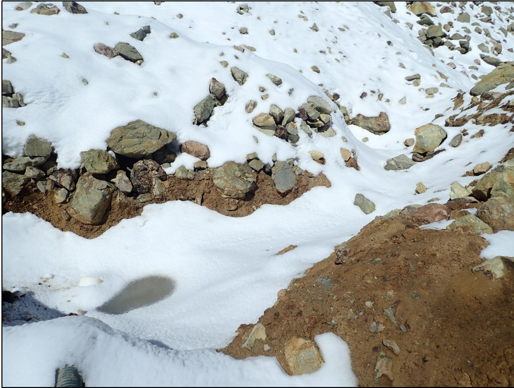
Photo 5. Northern seep collection area, sump inside of toe berm; looking southwest.
