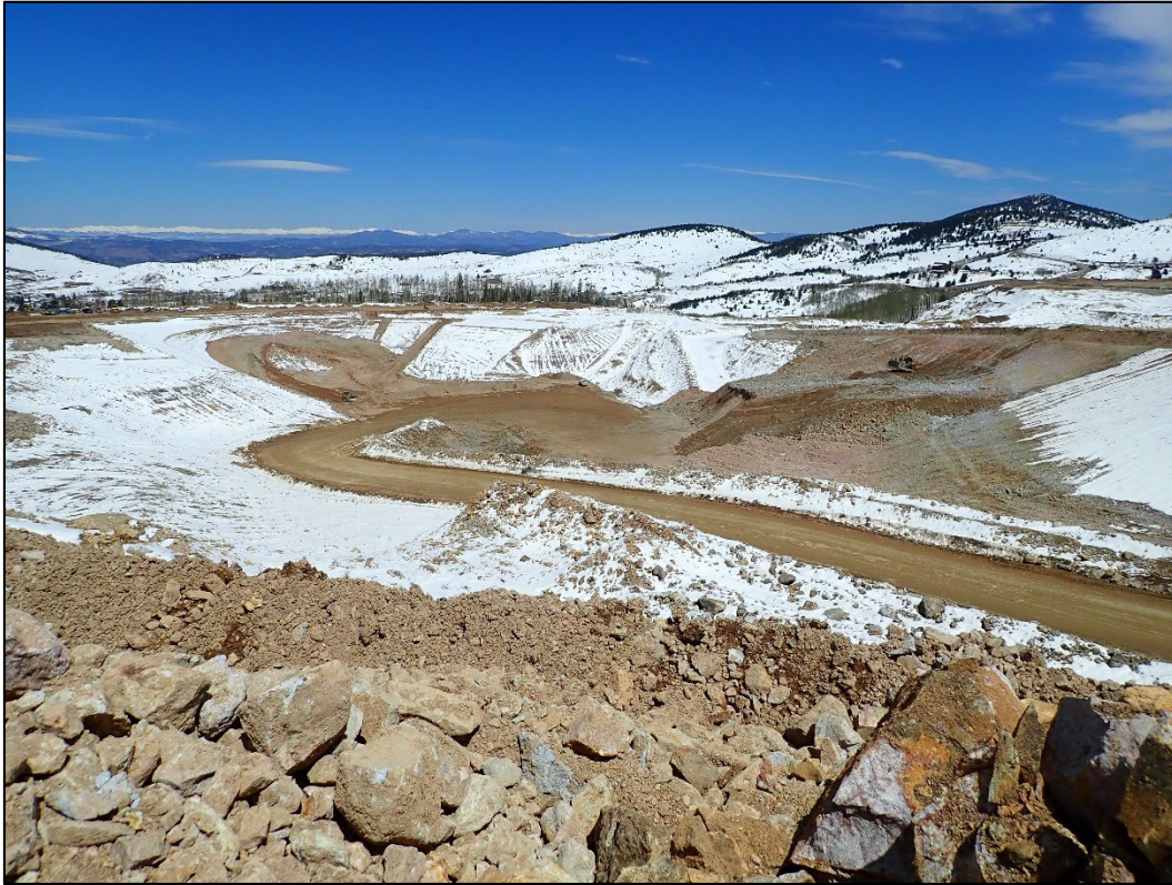
Photo 9. Schist Island Pit backfill area, Phase 3 VLF2 PSSA subgrade work occurring; looking northwest.
