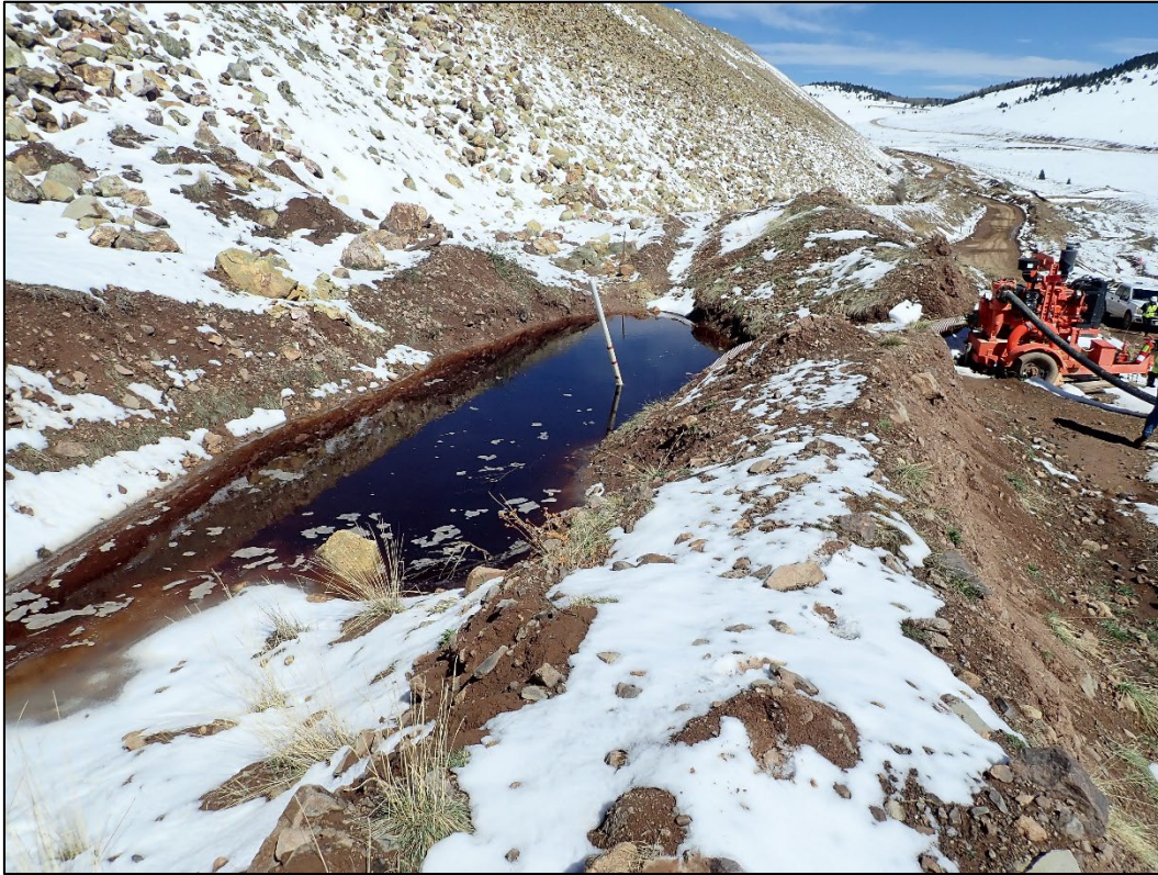
Photo 3. Southern seep collection sump; looking northwest.
