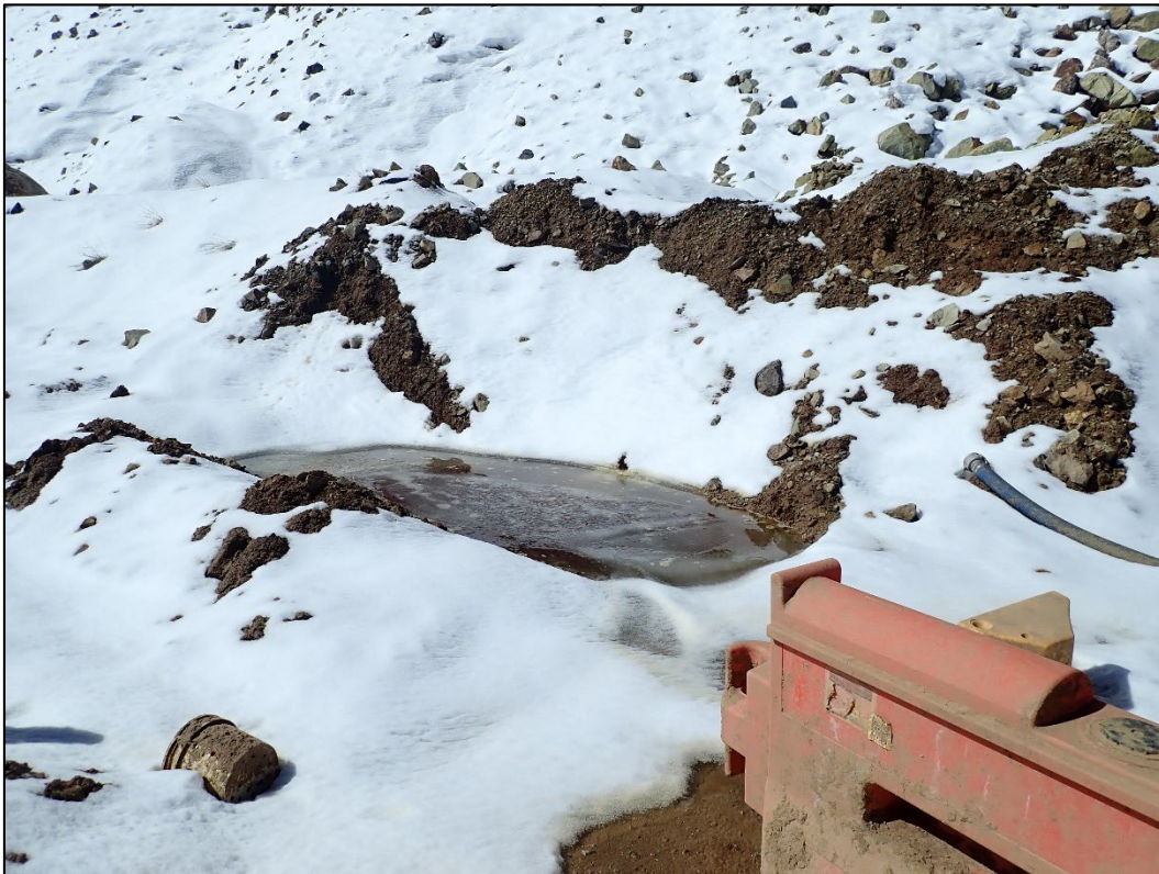
Photo 4. Northern seep collection area, sump outside of toe berm; looking southeast.
