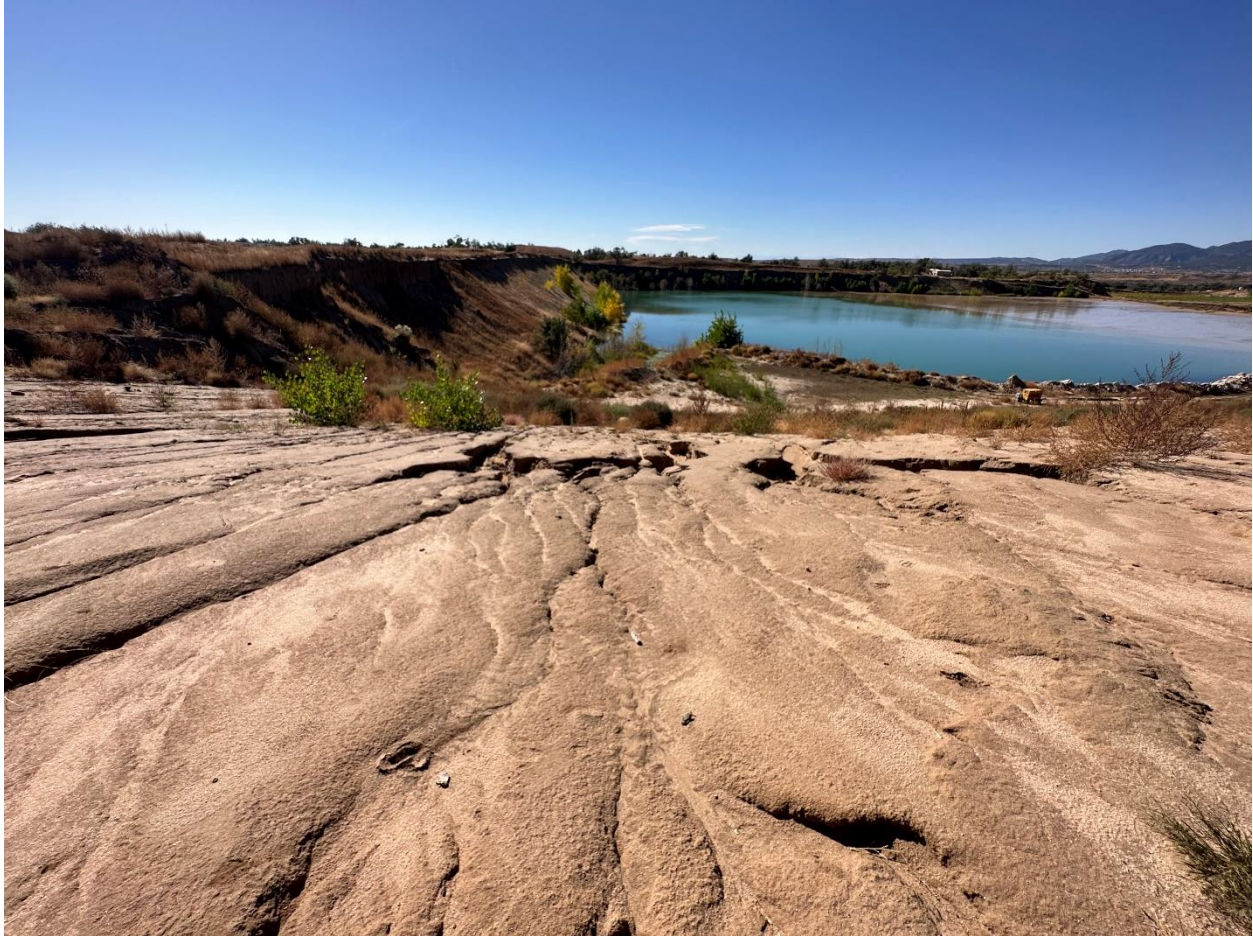
Photo 6. Buttress slope looking south, evidence of surface water drainage/erosion gully mid slope (eastern slope, less weeds)
