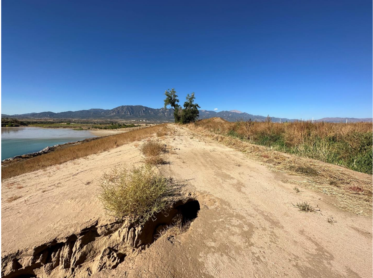
Photo 8. Erosion gully in relation to access road and ditch
