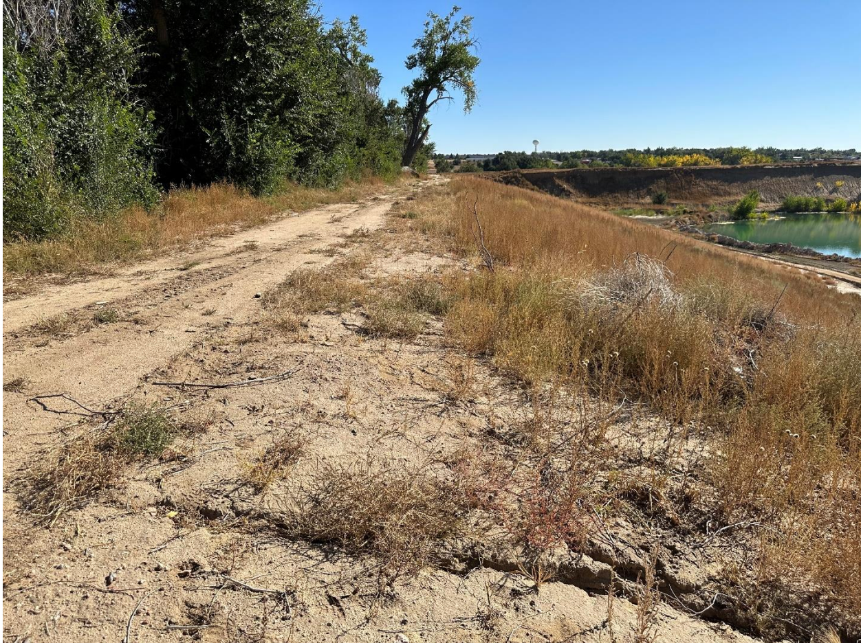
Photo 10. New surface drainage/erosion on access road (shallow), located middle alignment
