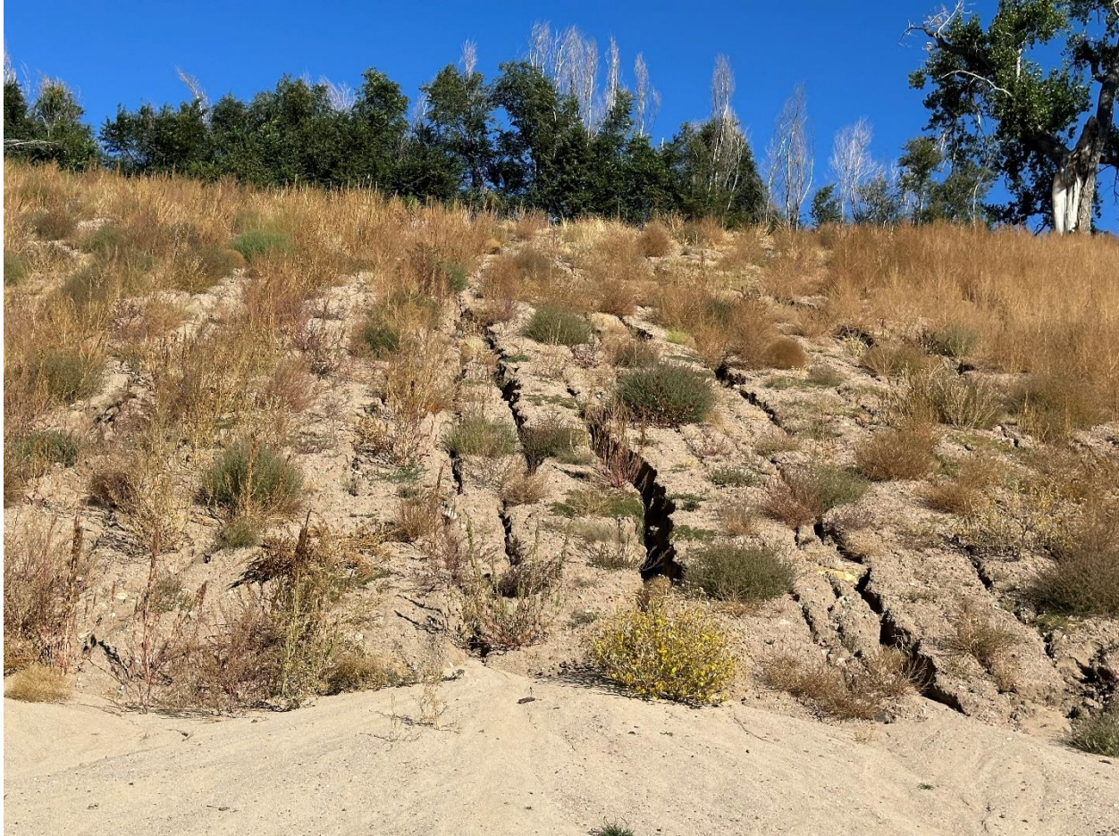
Photo 7. Buttress slope looking north, note expanding evidence of drainage/erosion gullies forming. More sediment near toe
