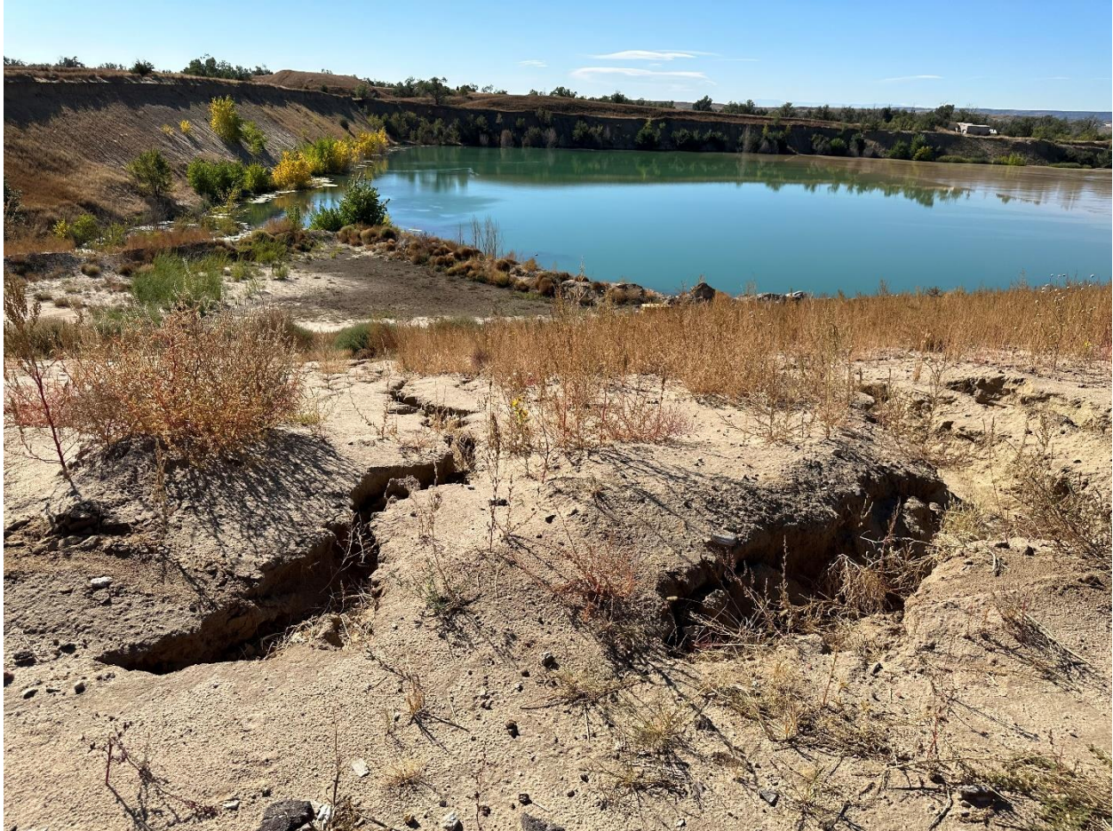
Photo 9. Zoomed in erosion gully south of access road (eastern slope)
