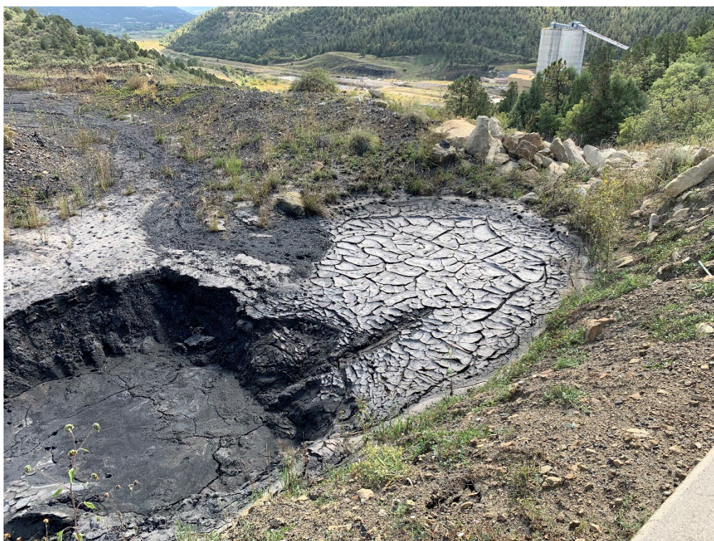
Photo 12 – Sediment trap on the RDA needs cleaning
