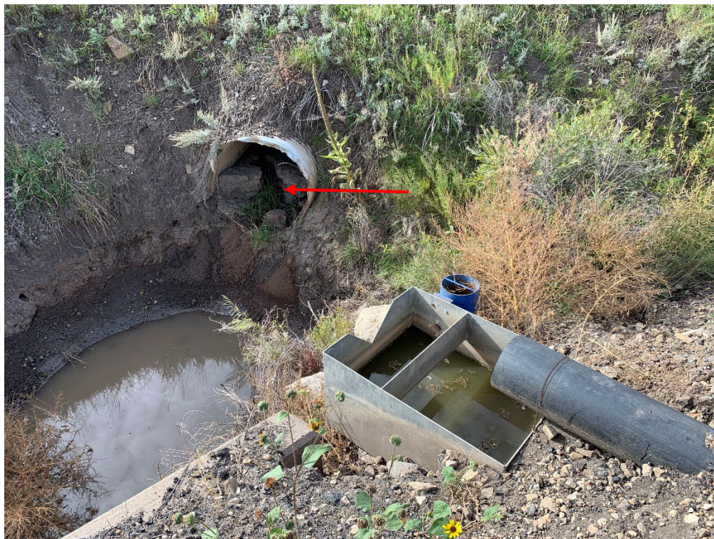
Photo 5 – Clean water culvert needs cleaning
