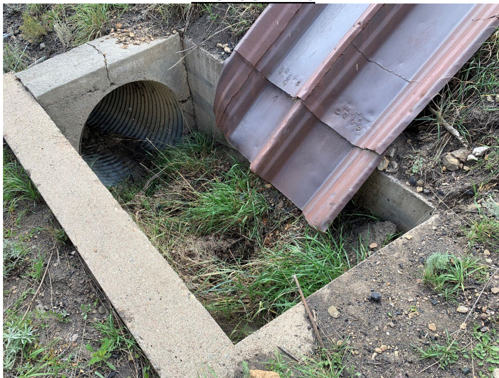
Photo 1 – Box at bottom of Ditch D26 flume
