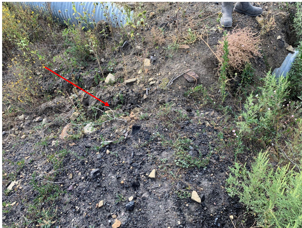
Photo 9 – Gullies forming on sediment basin berm
