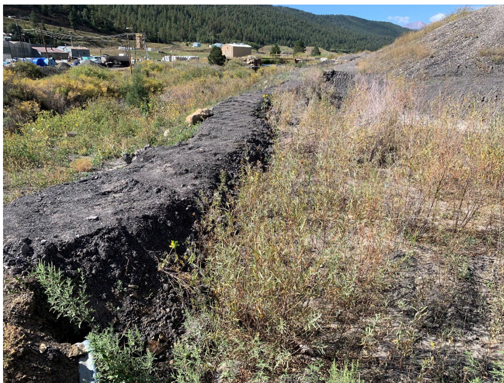
Photo 8 – Sediment basin berm needs sides sloped and compacted
