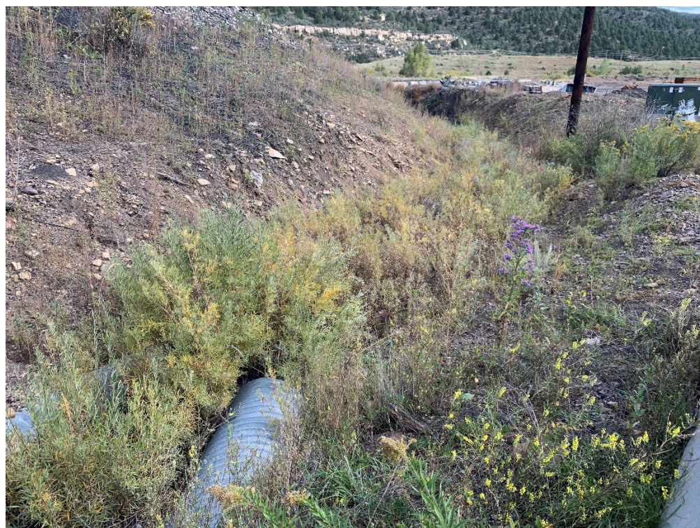
Photo 4 – Willows are impeding ditch flow
