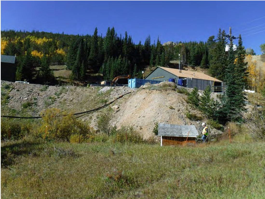
Photo 9: Water treatment plant
