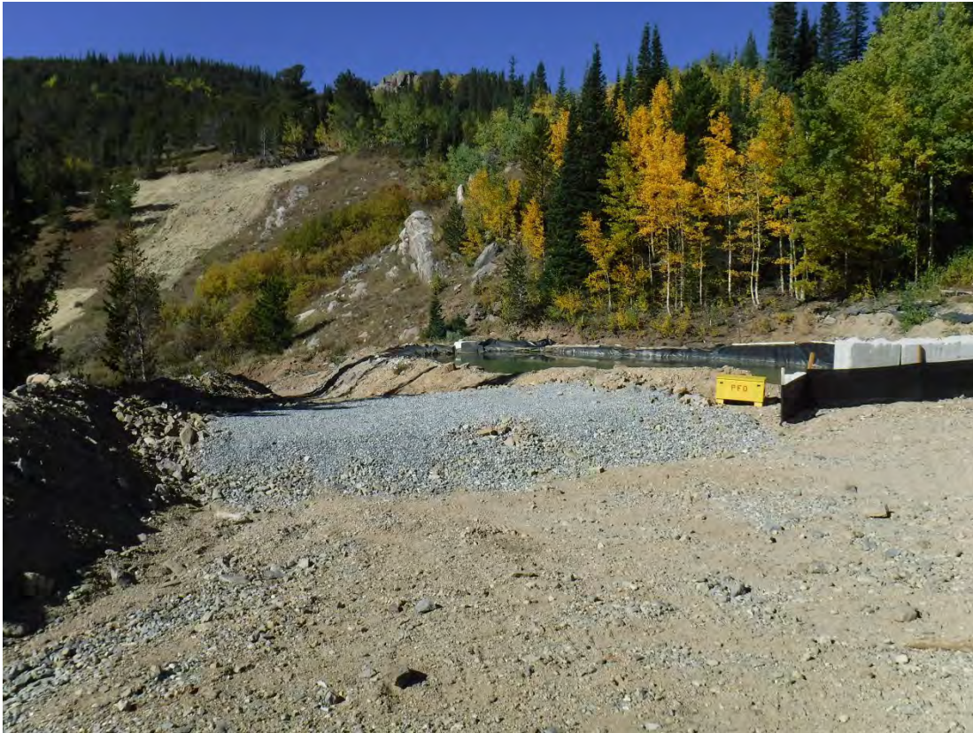
Photo 11: Rock check dam to aid in surface erosion control near Pond 3c
