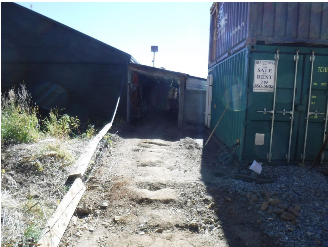
Photo 6: Snow shed and rail removal from the Cross Mine portal
