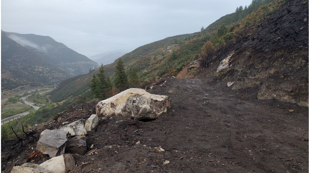
Figure 10: Top of new road, September 14, 2022
