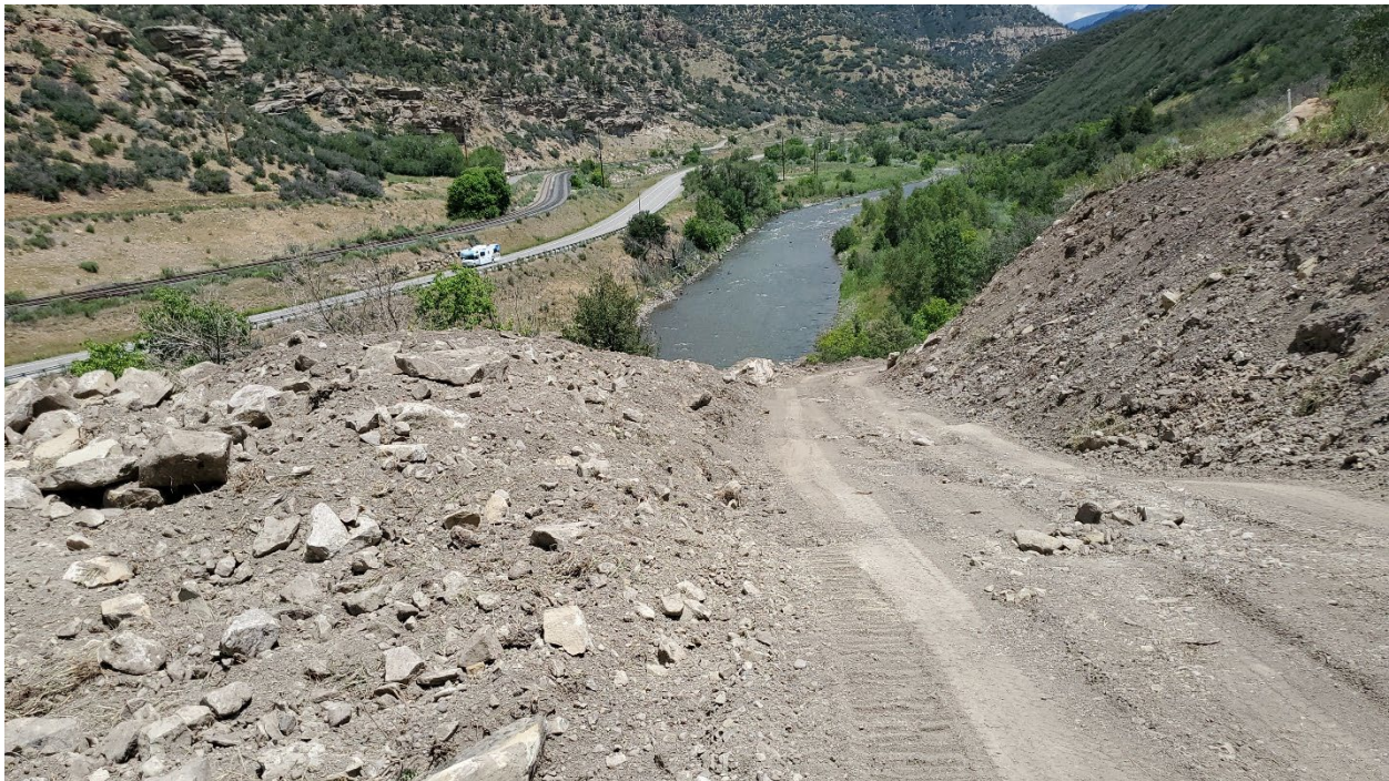
Figure 7: Partially constructed road, July 13, 2022
