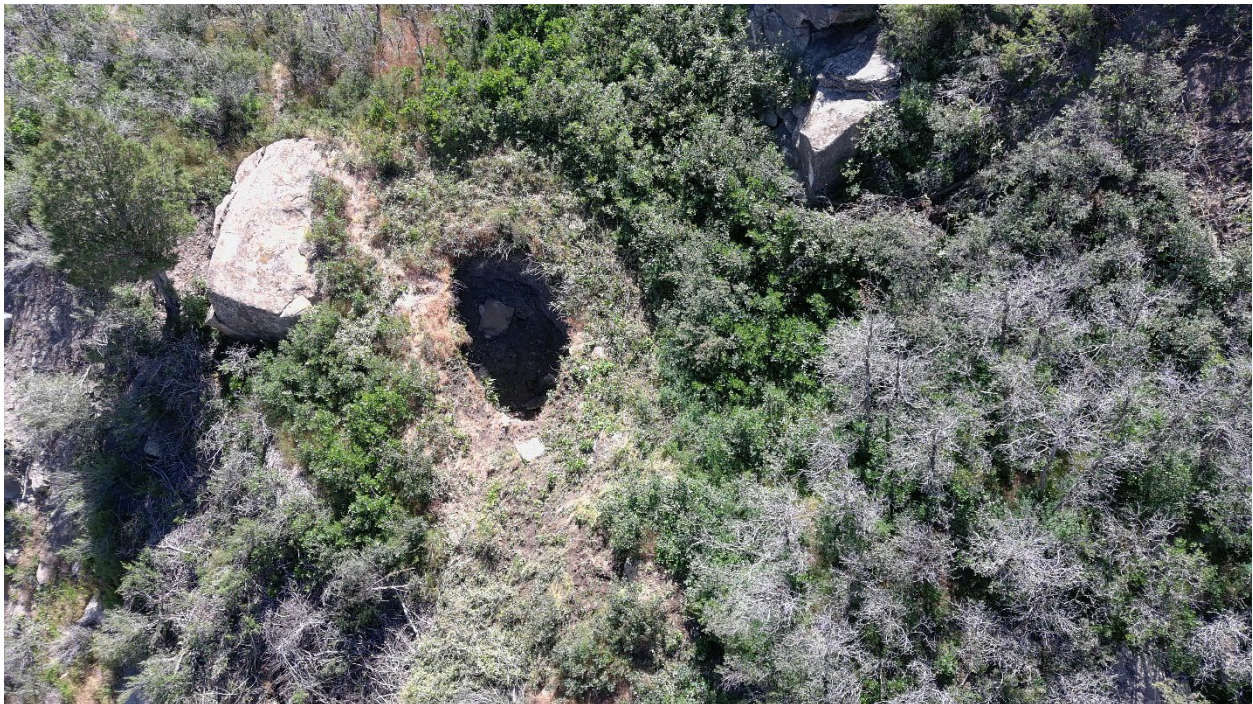
Figure 5: Close up of prominent vent, June 15, 2022
