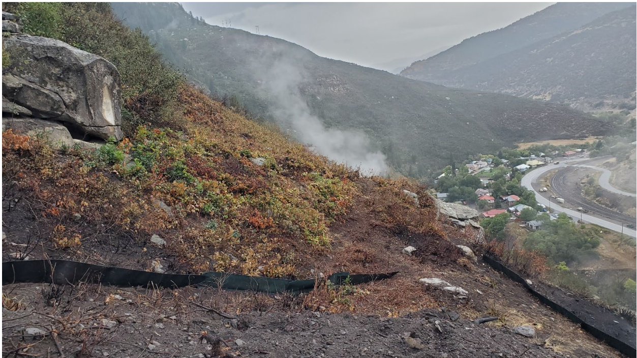
Figure 11: Sediment control in place, September 14, 2022
