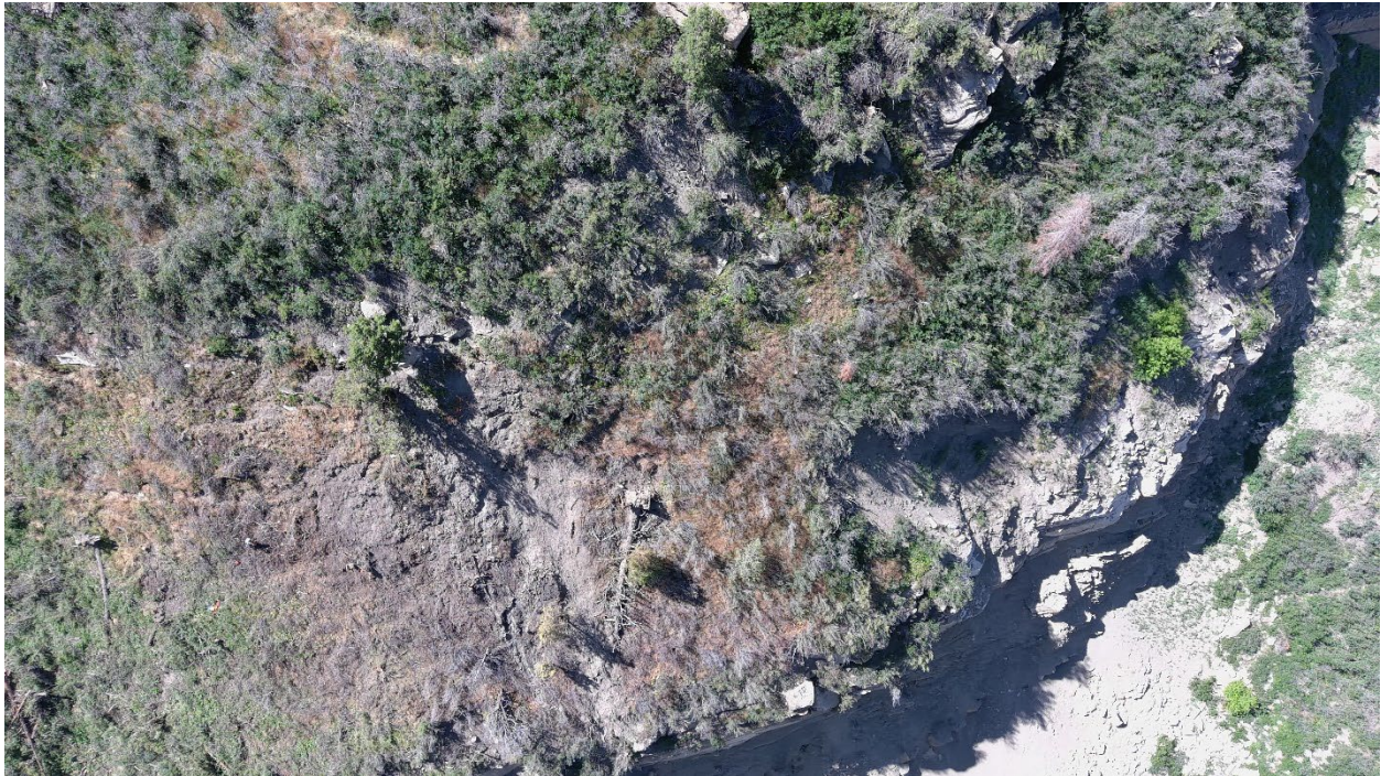
Figure 2: Aerial photo of mitigation work in progress, June 15, 2022
