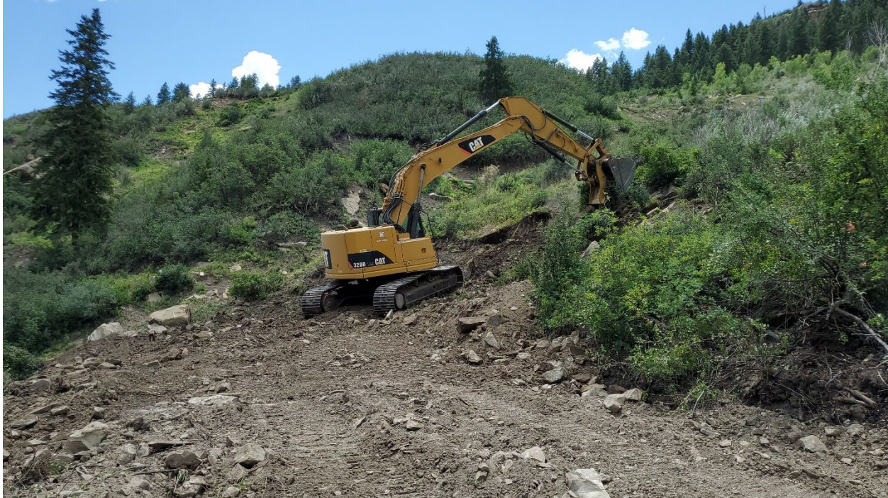
Figure 6: Road under construction, July 13, 2022
