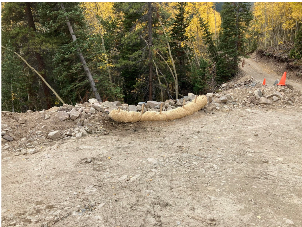
Photo 4 – Sediment control structure at pad area
