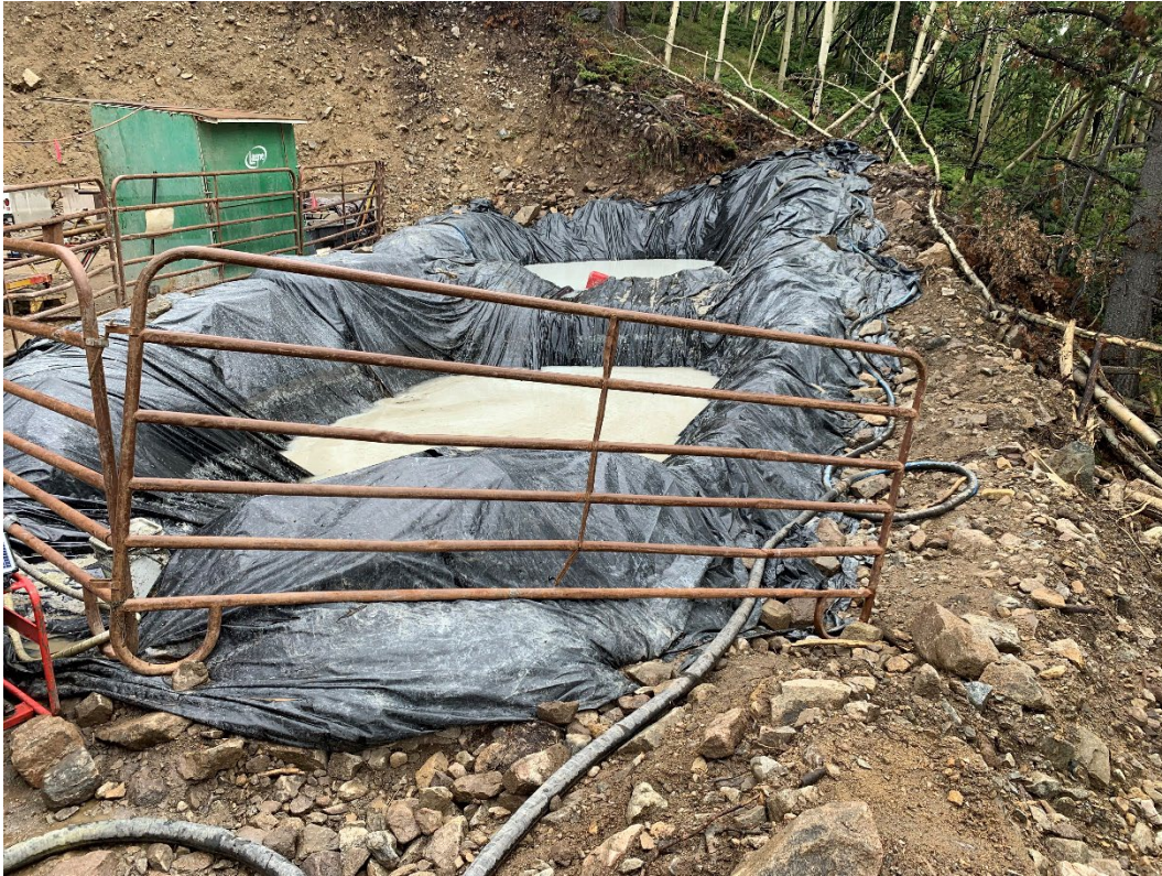
Photo 3 – Drilling fluid sumps
