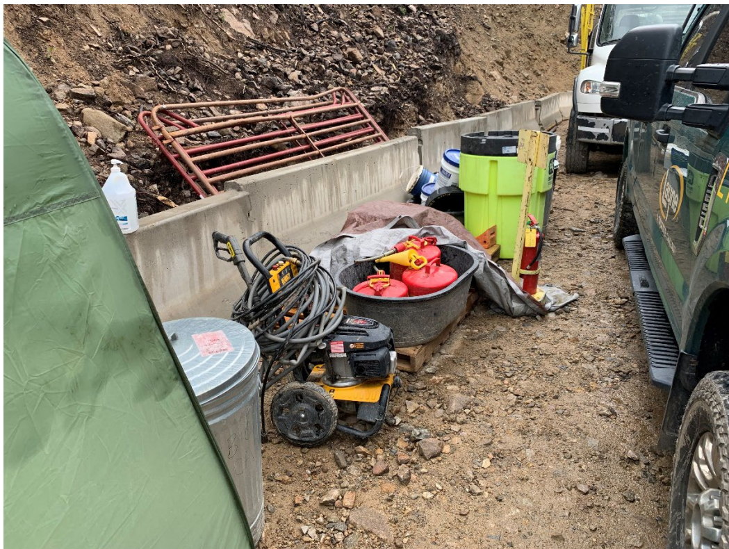
Photo 2 – Fuel storage secondary containment
