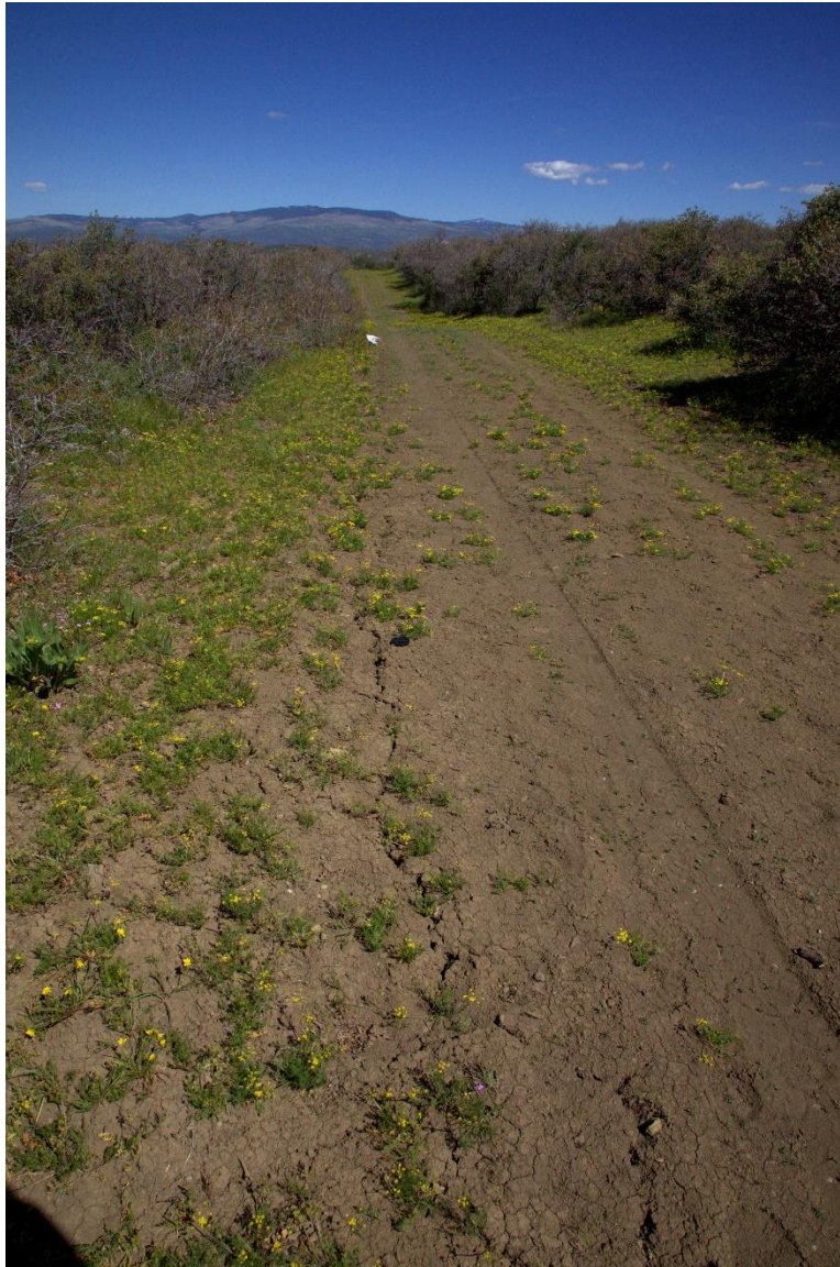
Figure 1: Southeast view of subsidence crack parallel to road on Traverse C-C' located over the E14 Headgate, between crosscuts 23 and 22.
