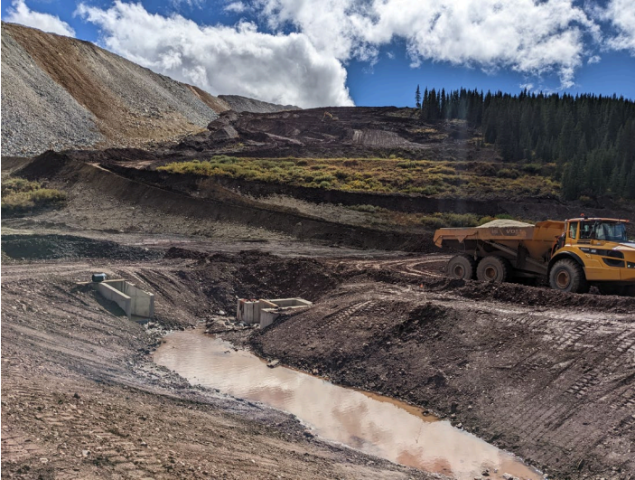
Topsoil being salvaged from the slope in the McNulty expansion area
