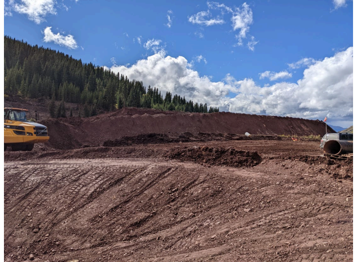
Topsoil stockpiled at base of McNulty expansion area
