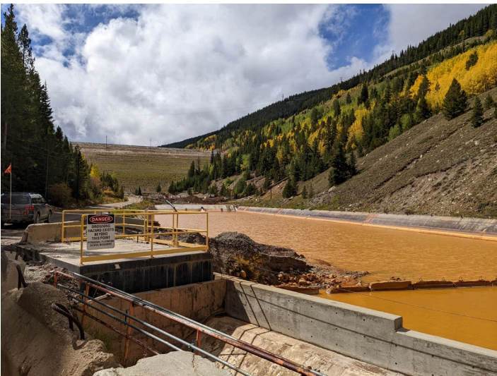
Concreted pond below 5 Dam
