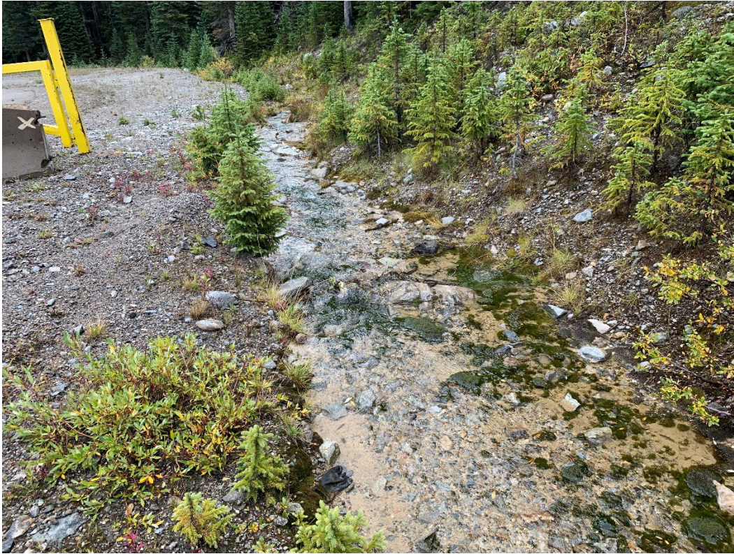
Photo 3 – Clear water diversion ditch
