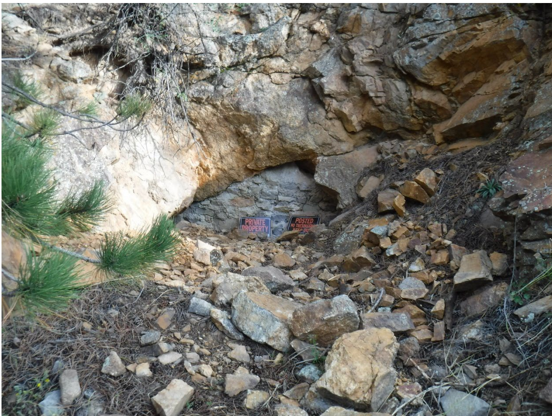
Photo 8: West Adit, Portal #7, note stone bulkhead
