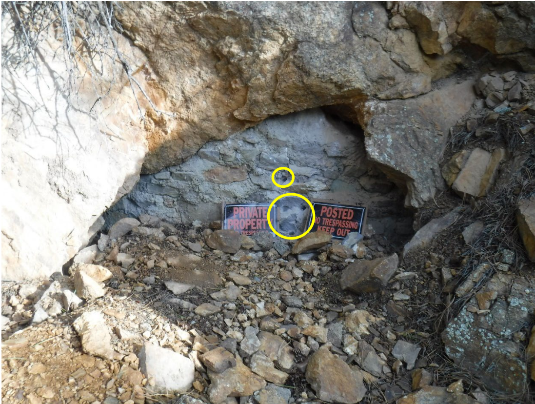
Photo 9: West Adit, Portal #7, shallow drill holes highlighted
