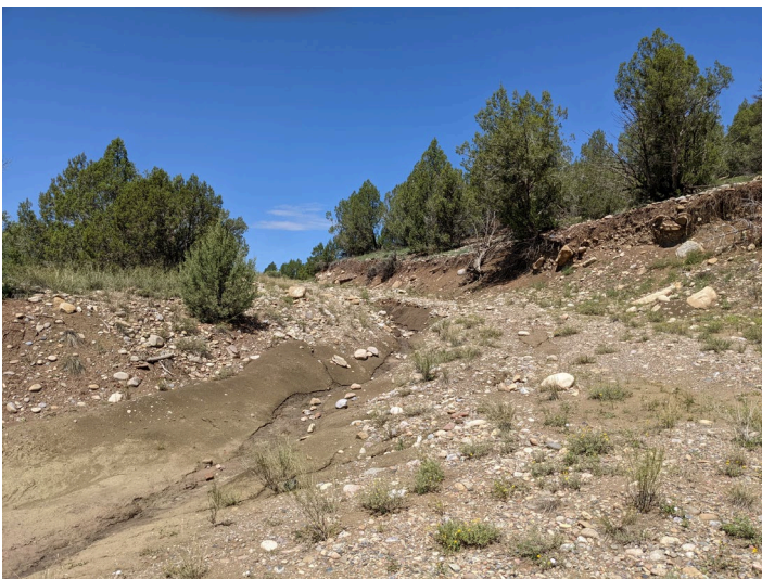
Access road erosion near scalehouse
