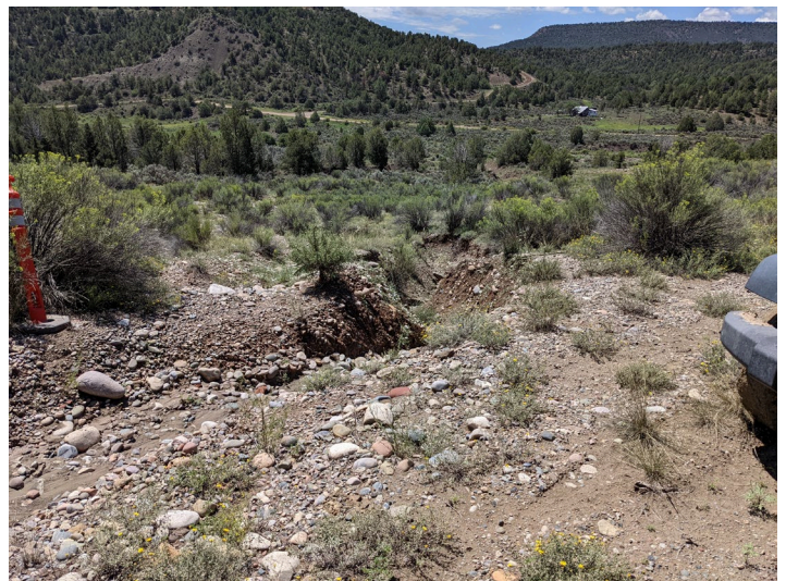
Access road erosion near scalehouse
