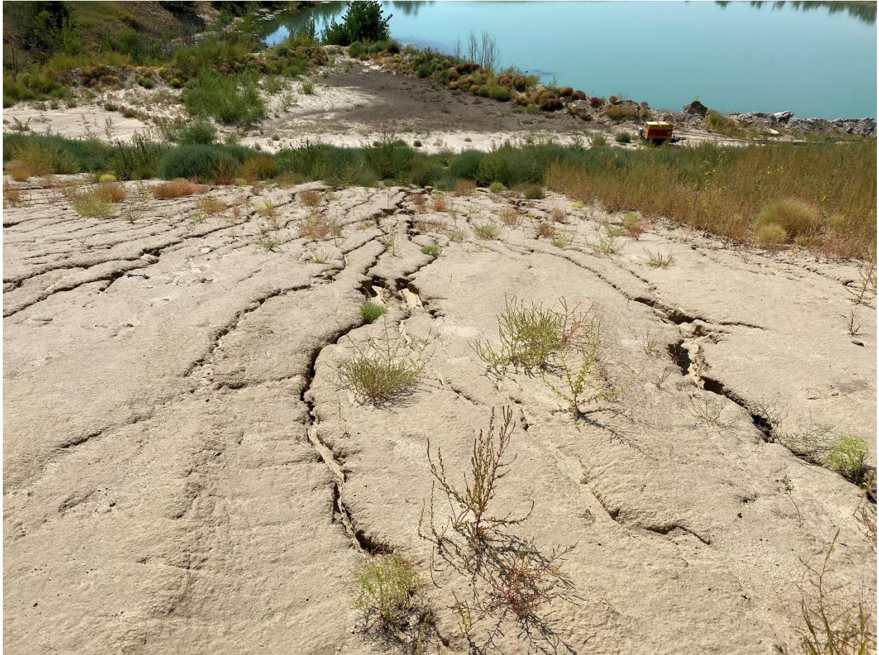
Photo 6. Buttress slope looking south, evidence of surface water drainage/erosion (eastern slope, less weeds)
