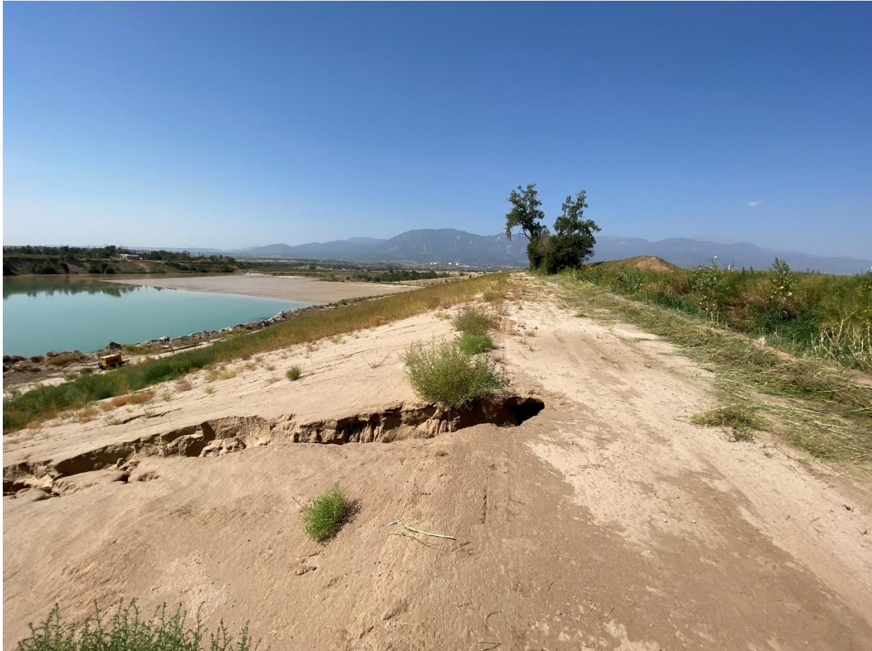
Photo 8. Erosion in relation to access road and ditch
