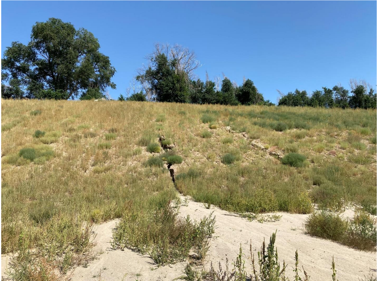
Photo 7. Buttress slope looking north, note expanding evidence of drainage/erosion forming
