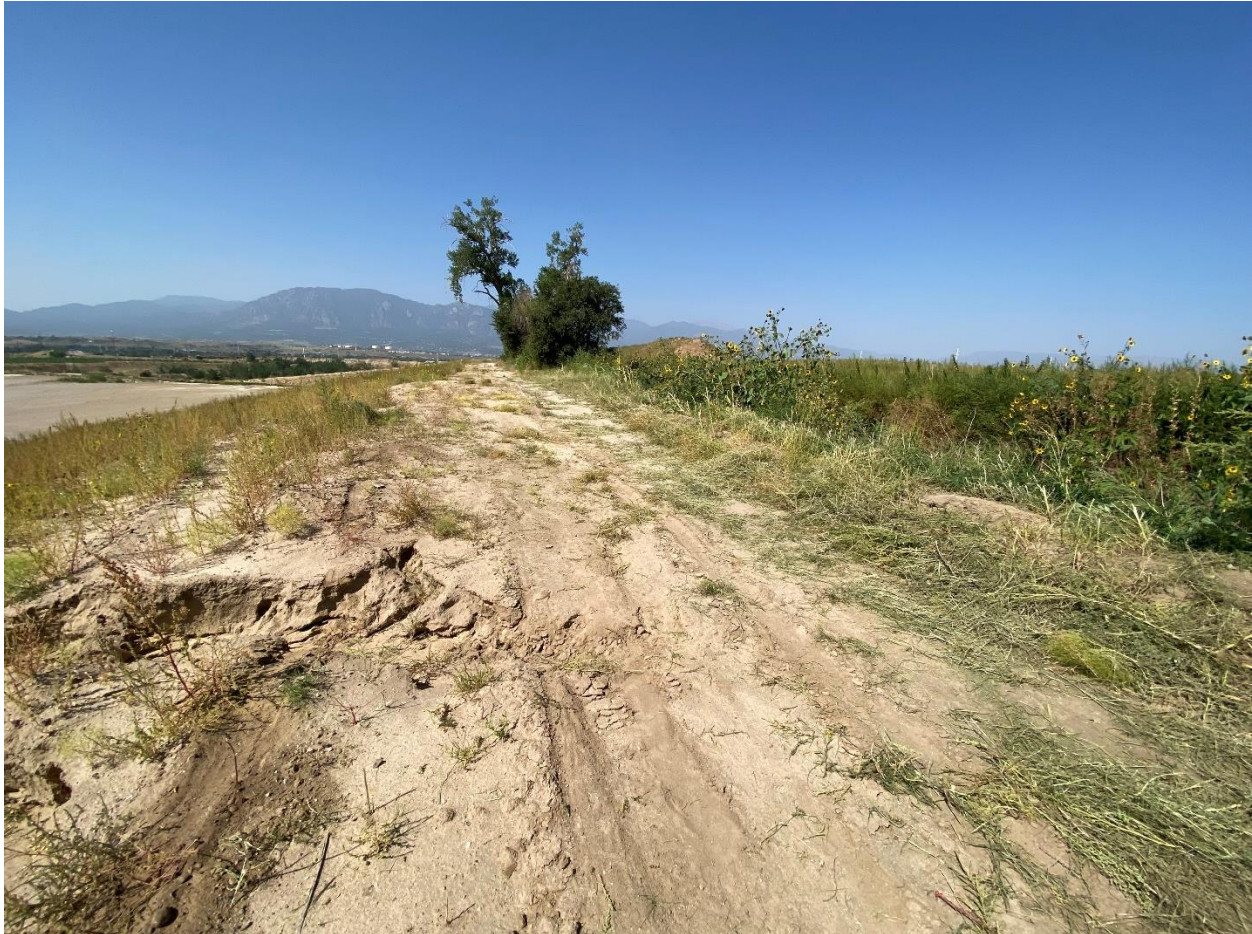
Photo 10. Second location of surface drainage/erosion on access road (shallower)
