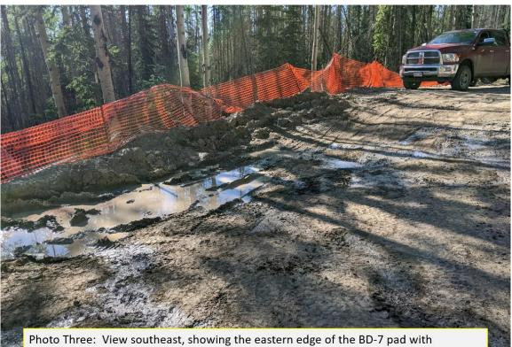
construction fencing and storm water control features that are functioning as designed.
