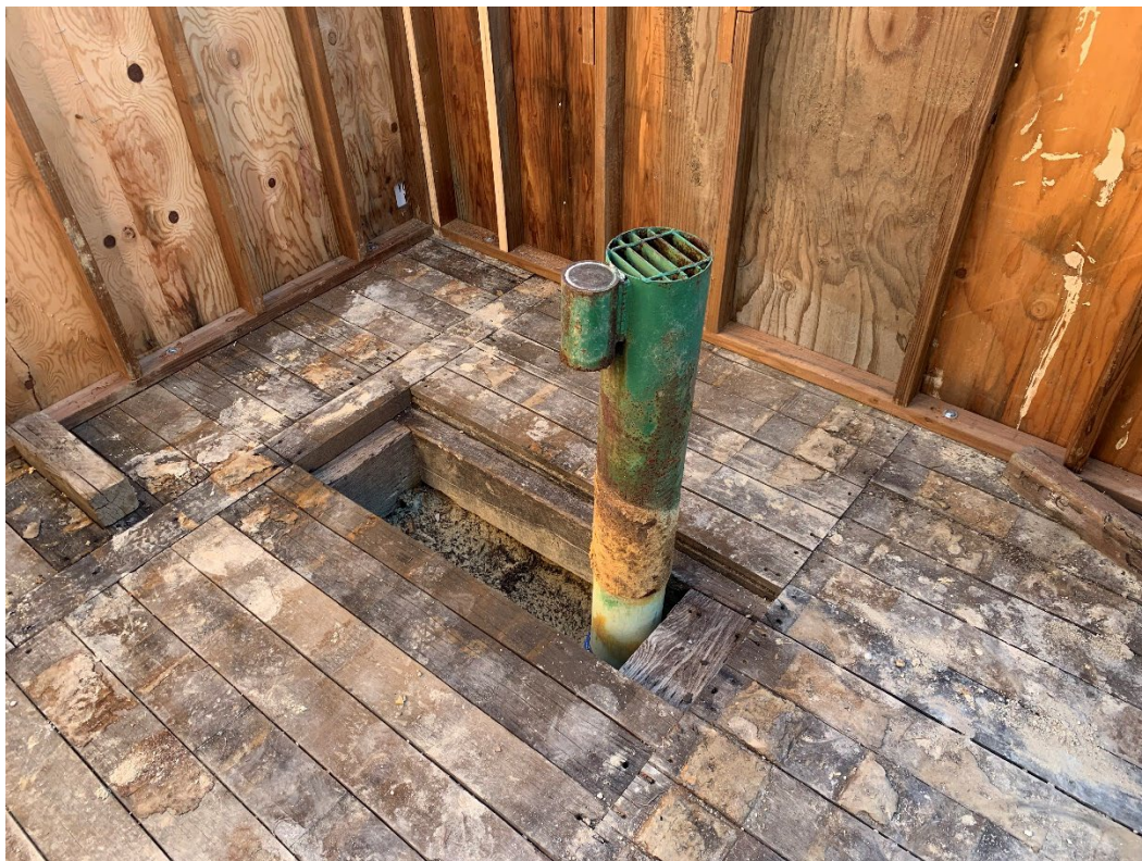
Photo 2 – Pipe identifying and venting the sealed mine shaft.
