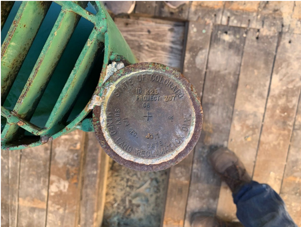
Photo 1 – Brass cap on shaft marker
