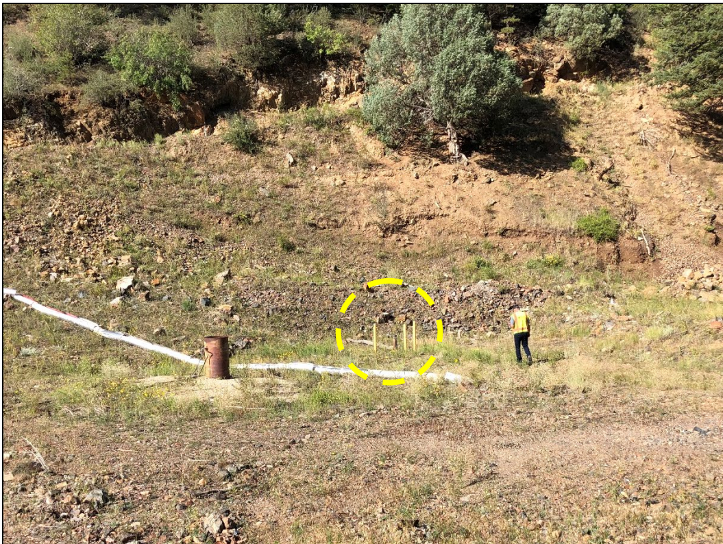
Photo 2. View looking south at groundwater monitoring well MW-18 (circled), installed at southern edge of valley (northwest of mesa with water treatment plant).
