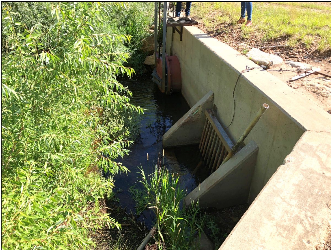
Photo 10. View of upgradient cutoff wall/headgate in Ralston Creek, showing creek flowing upstream of cutoff wall. Upgradient flows were being routed around the mine site via the bypass pipeline.
