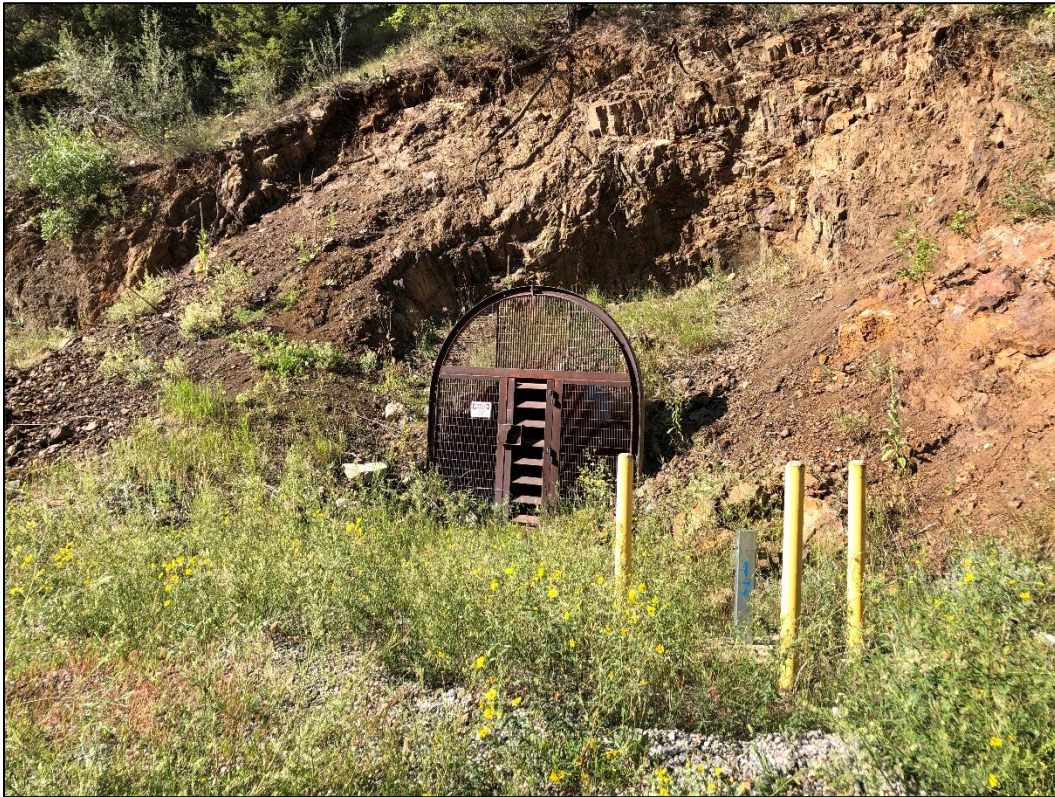
Photo 1. View looking south at groundwater monitoring well MW-17, installed near Pierce Adit (along road to mesa with water treatment plant).
