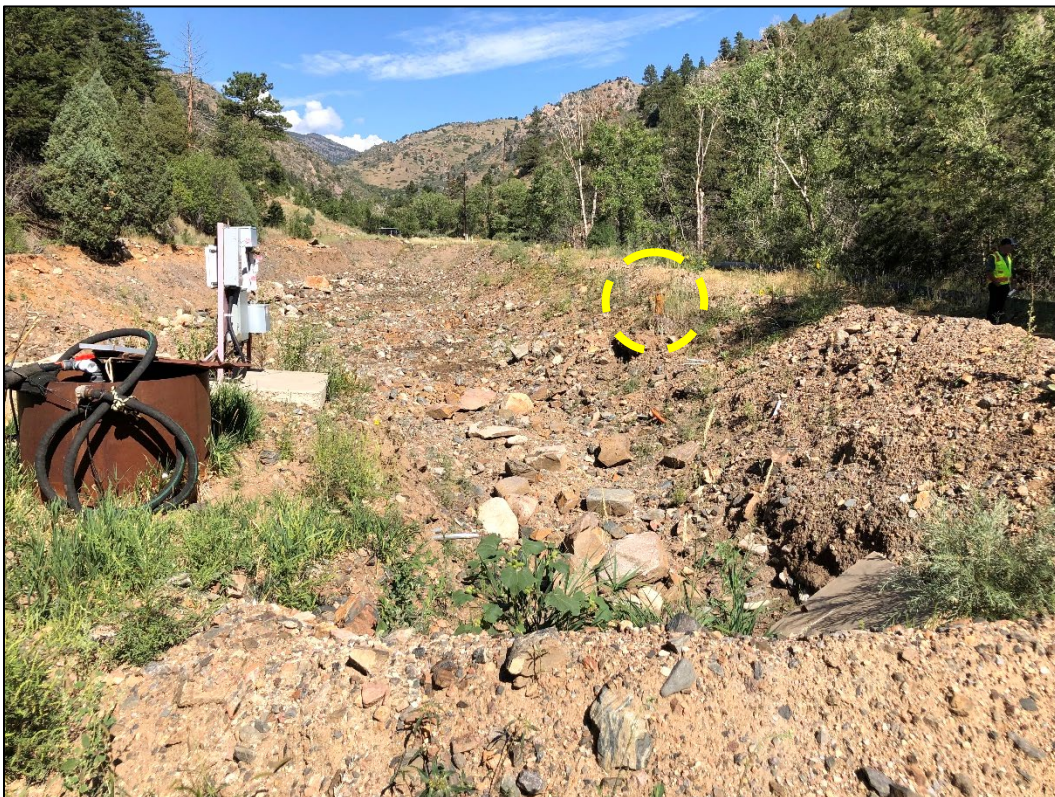
Photo 12. View looking northwest across southern portion of valley excavation project. Note master sump #1 and monitoring well MW-7 (circled) installed in this area. These features have been rendered inoperative due to the excavation project and will need to be removed from the monitoring plan.
