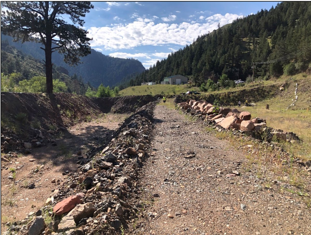
Photo 4. View looking southeast across central portion of valley excavation project. This project has been suspended since December 2021.
