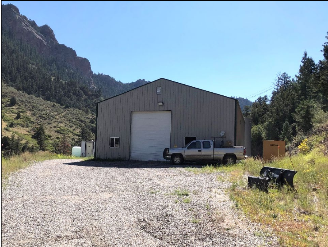
Photo 13. View looking southeast at northwestern side of water treatment plant (on top of mesa).
