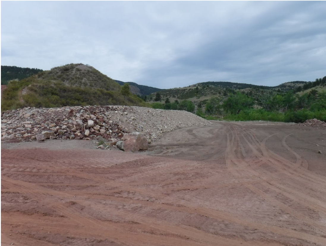
Photo 3: Scour berm in place, partially complete
