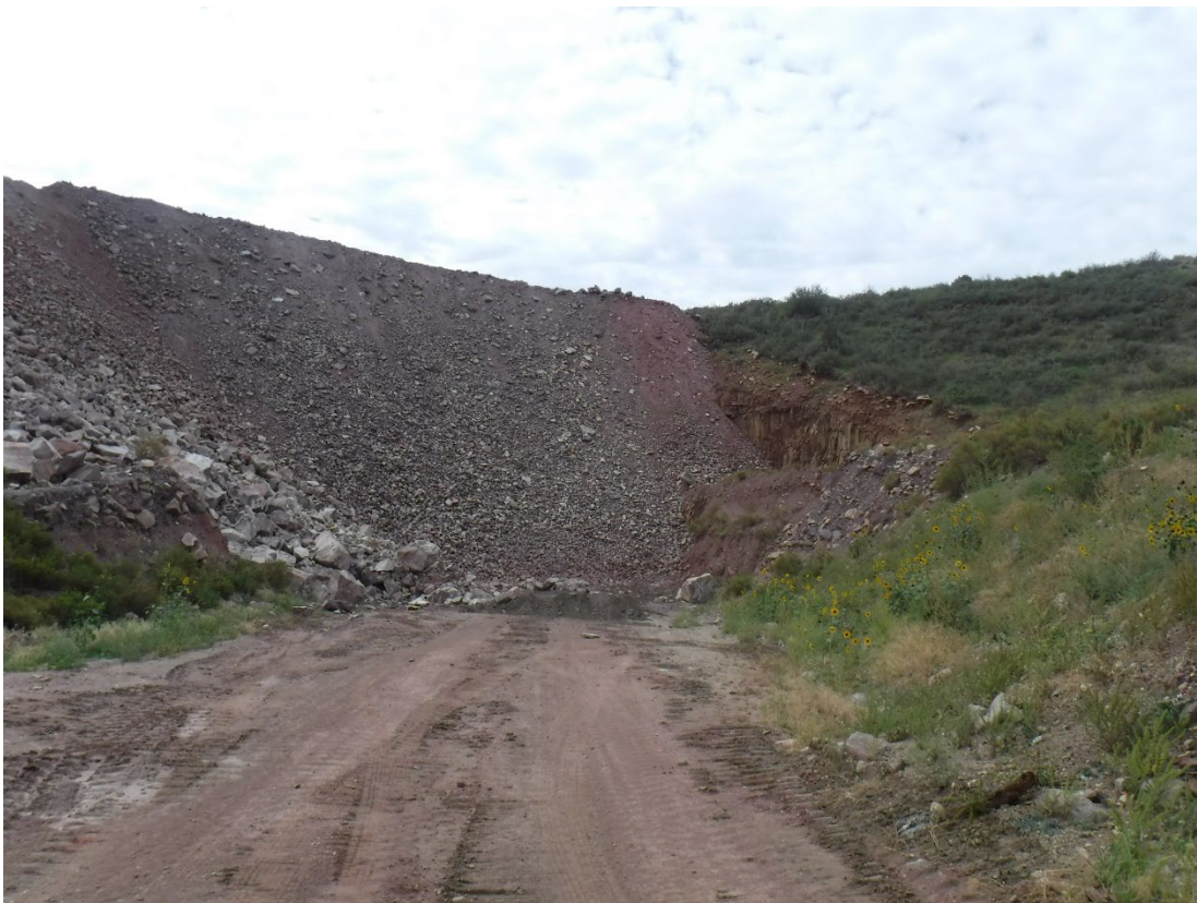
Photo 4: Quarry area 2 backfill progress, ~50% complete
