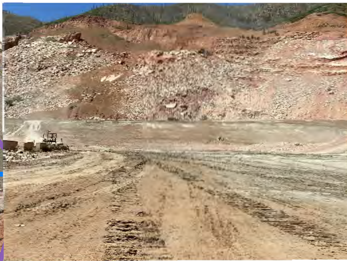
2. View of elevation change in pit floor - about 26 feet.
