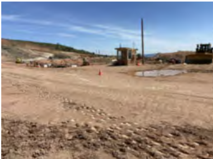
1. Shop was demolished and total station was relocated.
