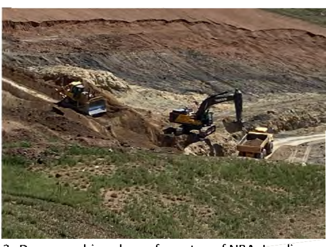
3. Dozer pushing down from top of NBA. Loading material and hauling to buttress area.
