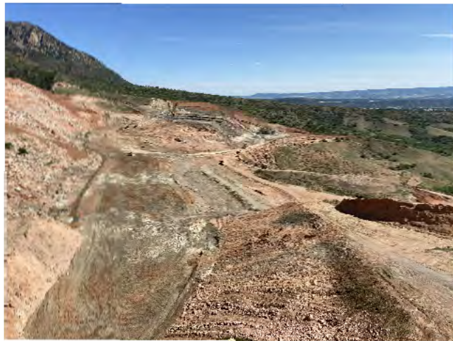
6. Compacted area in the pit looking north.
