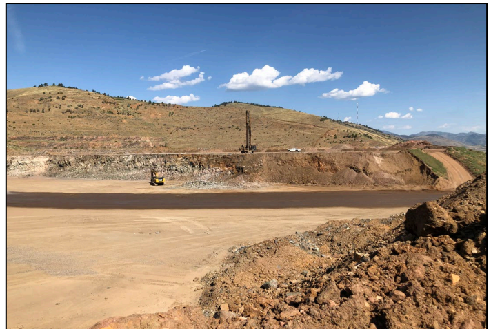
Photo 4 – Drilling for next blast in material removal area
