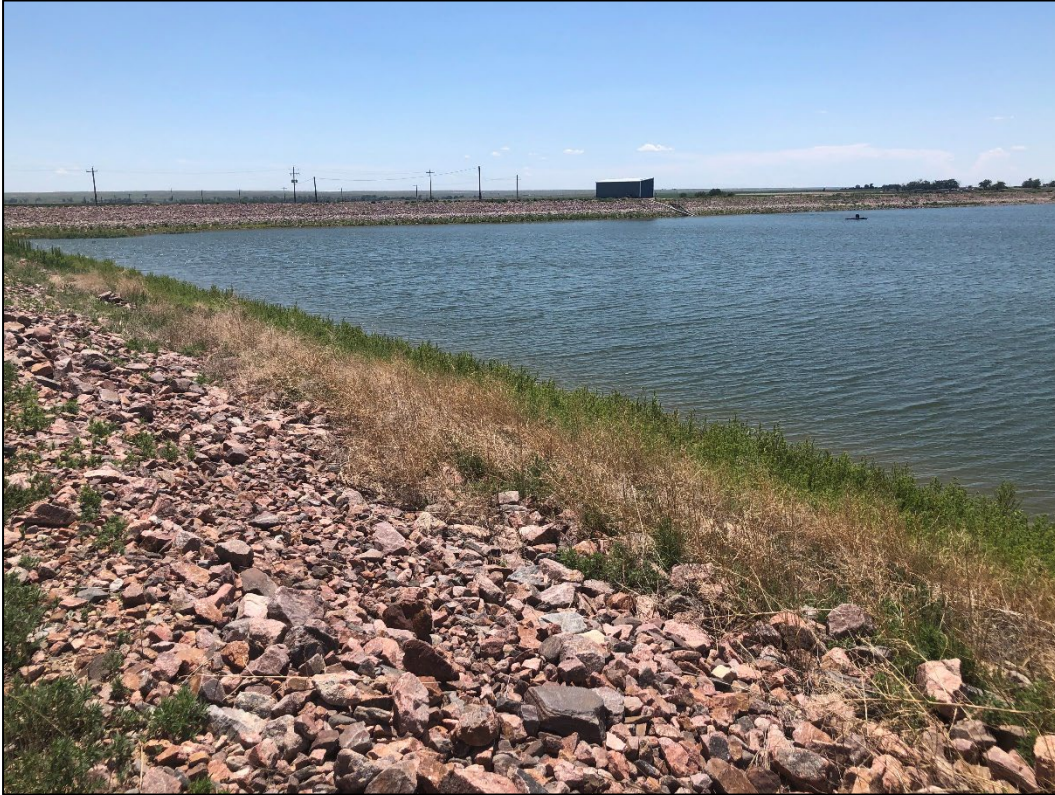
Photo 3. View looking southwest across southeastern portion of reservoir, showing riprap lined eastern (foreground) and southern shorelines.
