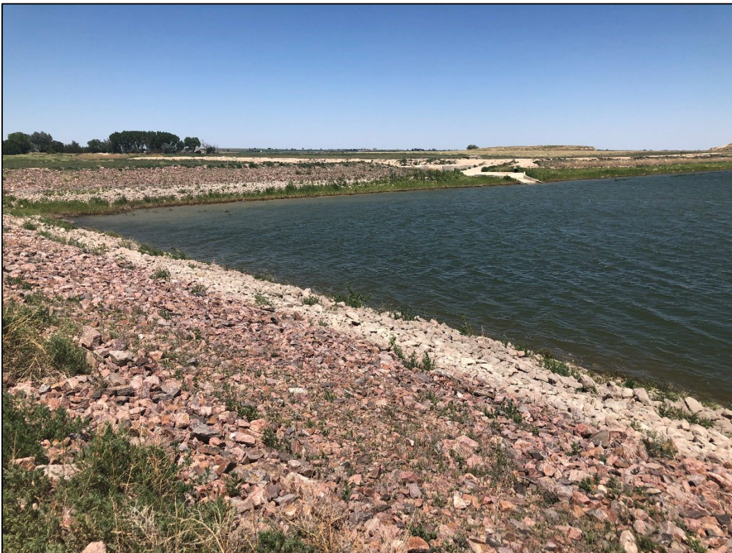
Photo 10. View looking northeast across northwestern portion of reservoir, showing riprap lined western (foreground) and northern shorelines.
