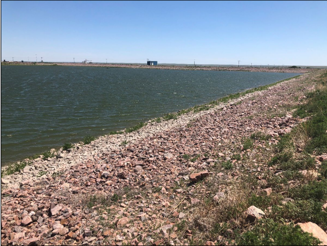
Photo 9. View looking southeast across southwestern portion of reservoir, showing riprap lined western (foreground) and southern shorelines.
