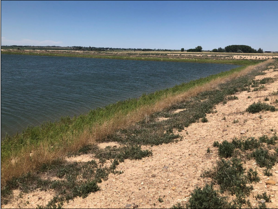
Photo 5. View looking northwest across northeastern portion of reservoir, showing portions of shorelines with no riprap and very little vegetative cover besides annual weeds (e.g., kochia, russian thistle).
