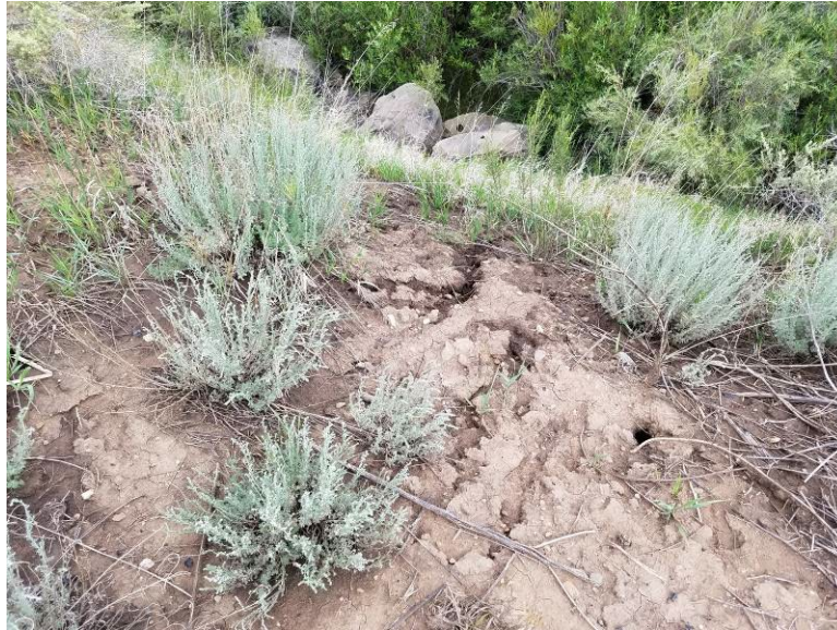
Figure 1. Pond 007a northern embankment, rill forming.
