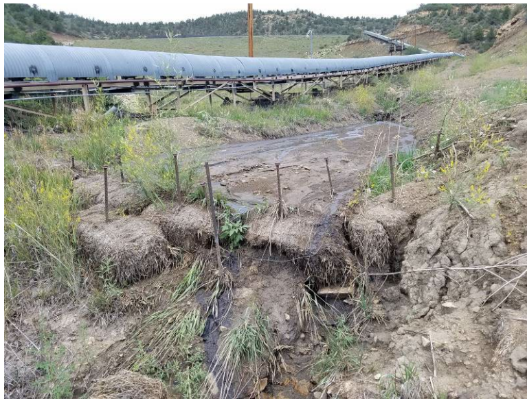
Figure 3. Straw check dam in drainage above Containment Area #5, east of the Conveyor.
