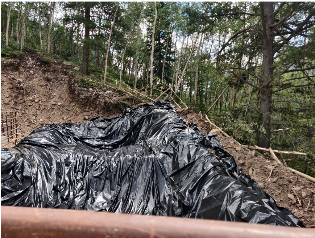
View of the triple lined mud pit
